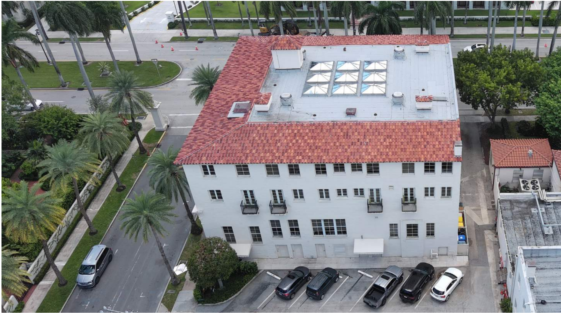
EXISTING PHOTO - NORTH ELEVATION
