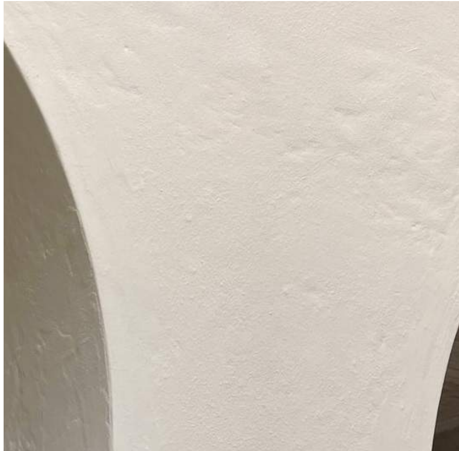
TEXTURED STUCCO - EXTERIOR WALL SURFACE, OTHER TRIM (RUN STUCCO)
