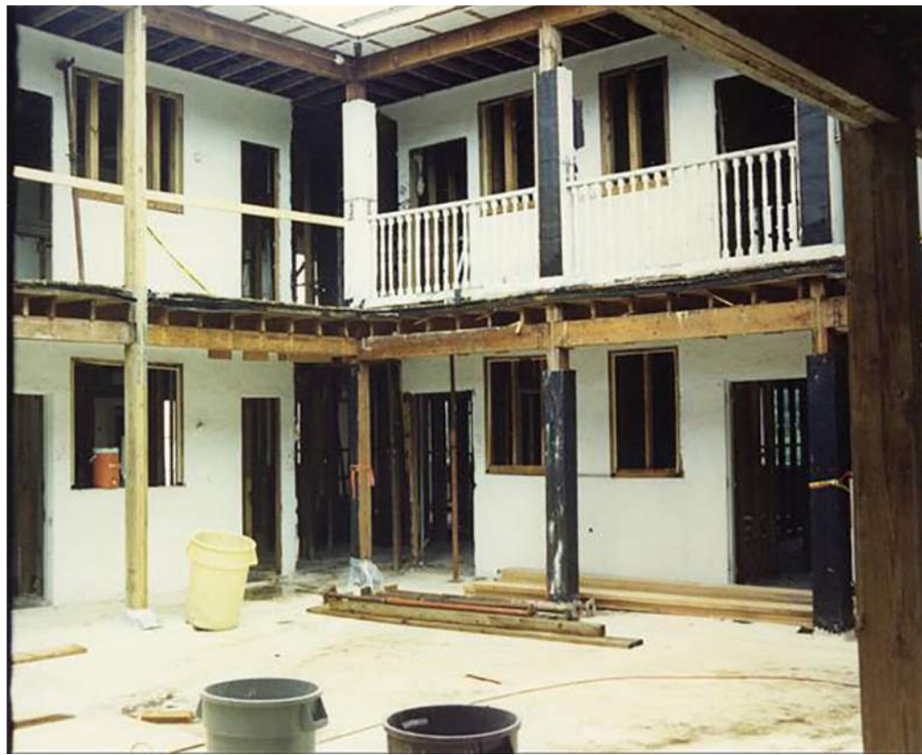
3 PHOTO - COURTYARD PRIOR TO DEMOLITION, 1992
