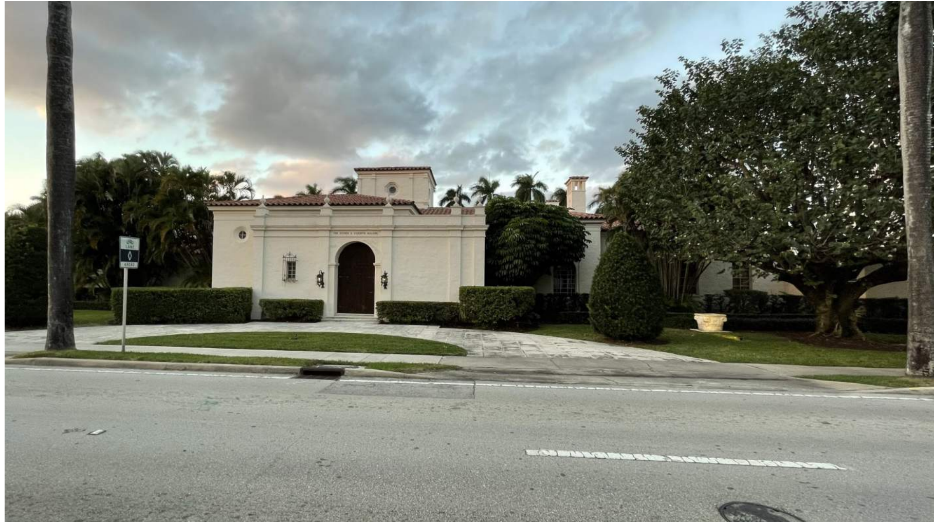
EXISTING PHOTOS - SOUTH ELEVATION
