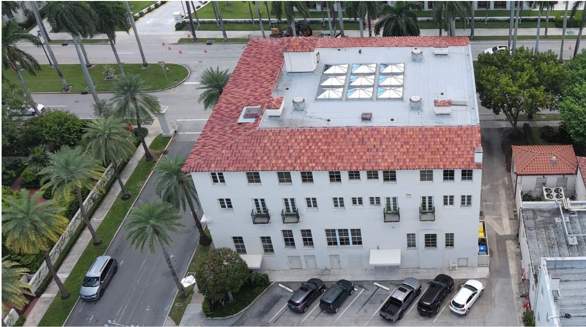
EXISTING PHOTO - NORTH ELEVATION
