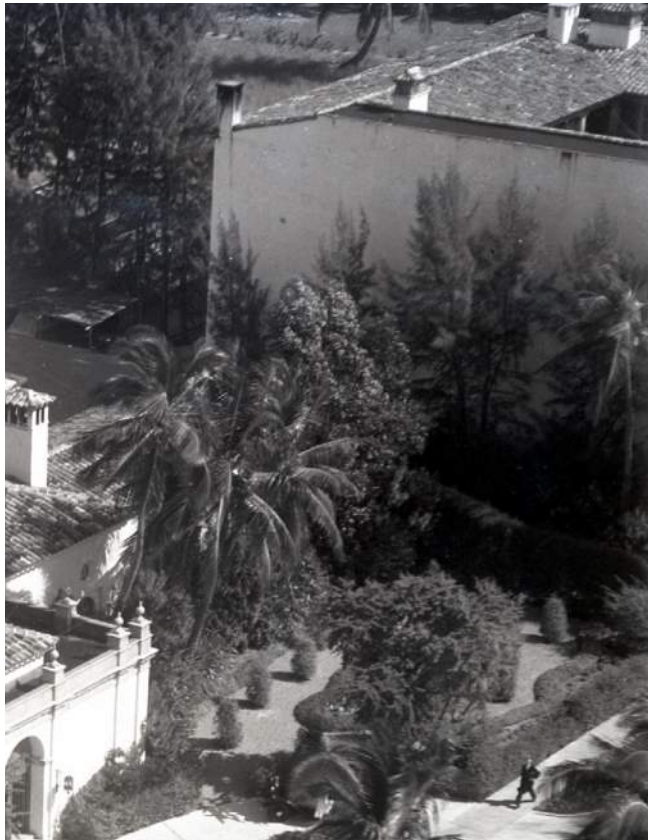
HISTORIC AND EXISTING PHOTO - WEST ELEVATION
