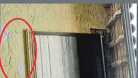
DIAGONAL CRACK IN THE TERRACOTTA WALL UNDER WINDOW SILL LOOKING FROM OUTSIDE
