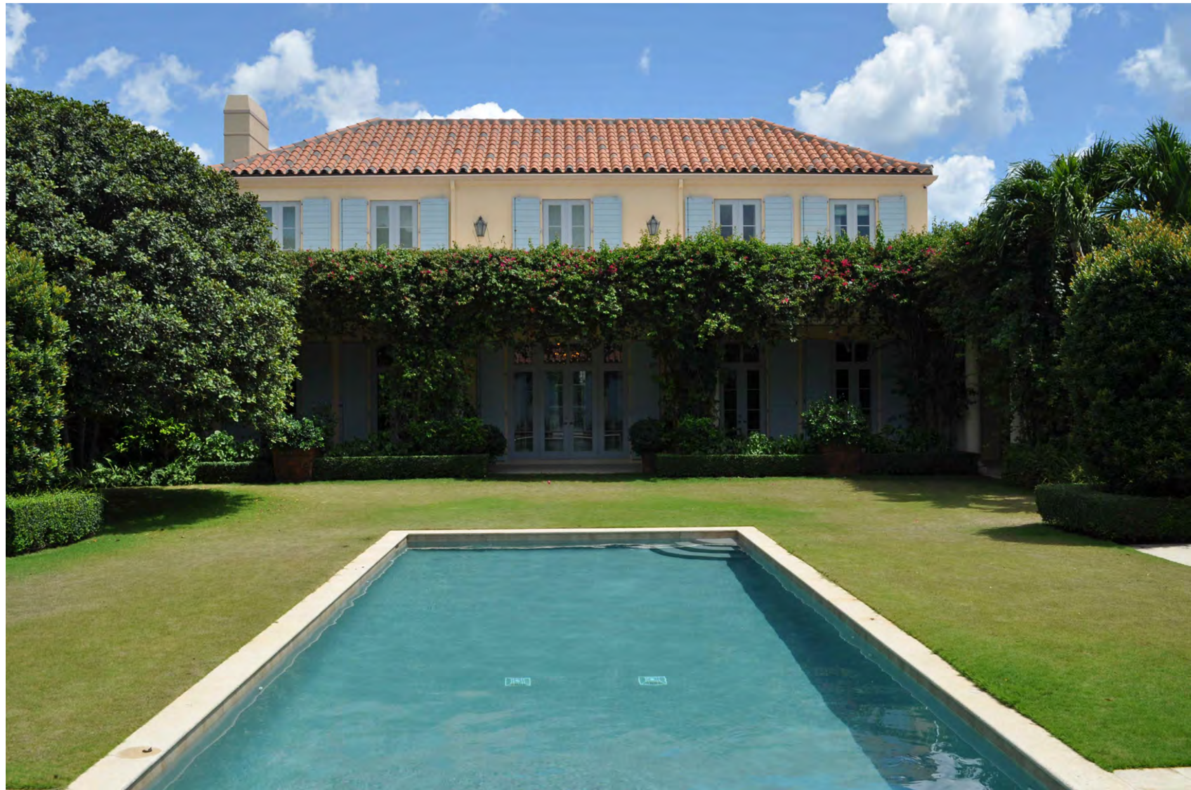
Existing Main House Rear Facade
