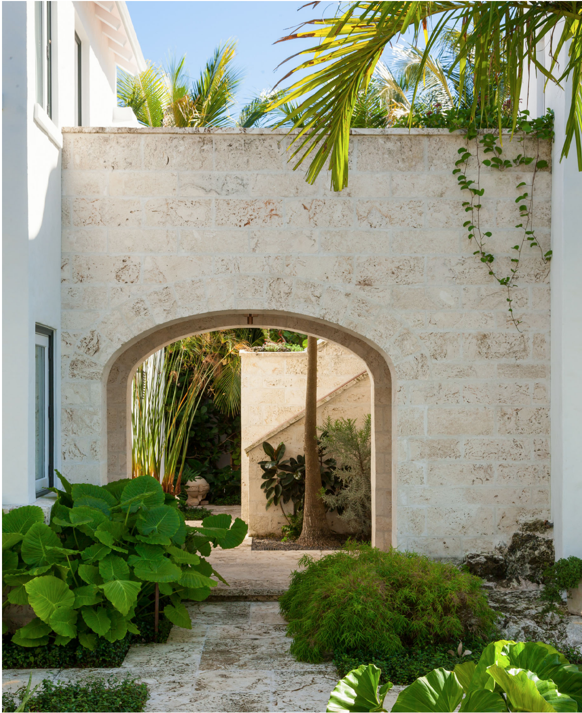
320 ISLAND ROAD GUEST HOUSE ENTRY
