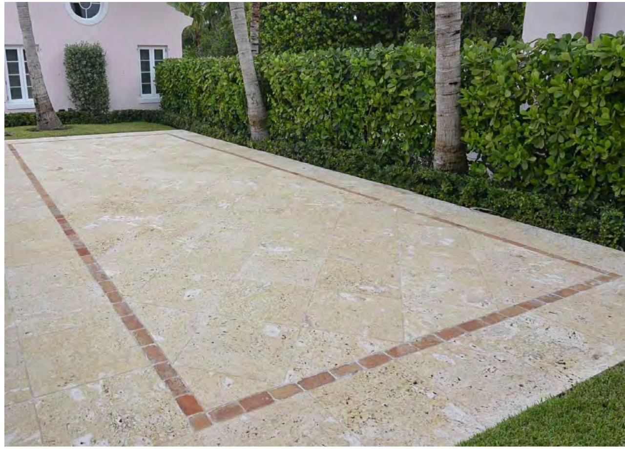
DOMINICAN SHELL STONE TERRACE WITH OLD CHICAGO BRICK INLAYS
