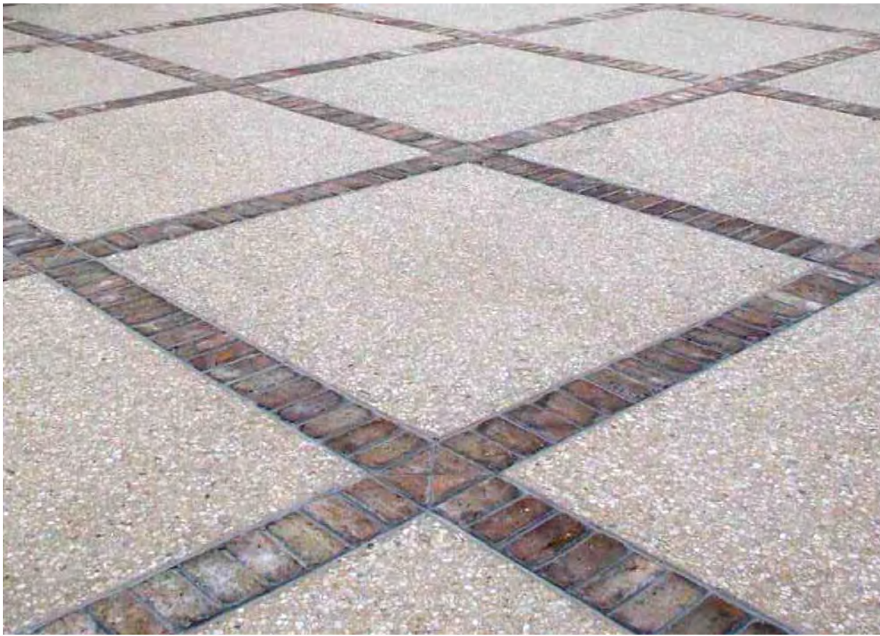
TABBY MOTOR COURT WITH OLD CHICAGO BRICK INLAYS
