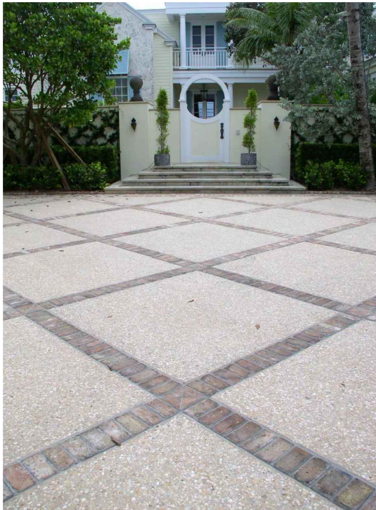
TABBY MOTOR COURT WITH OLD CHICAGO BRICK INLAYS
