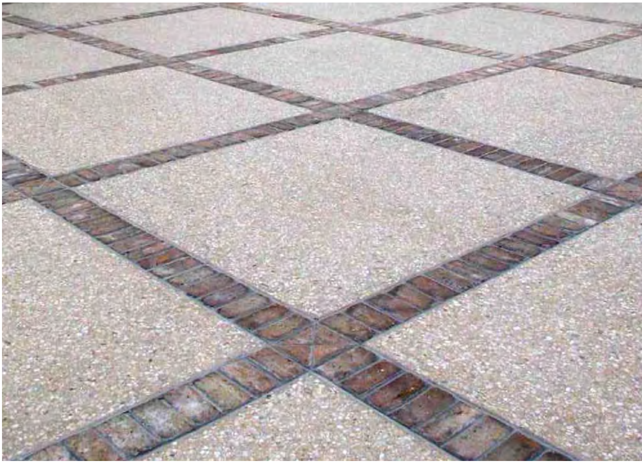
TABBY MOTOR COURT WITH OLD CHICAGO BRICK INLAYS
