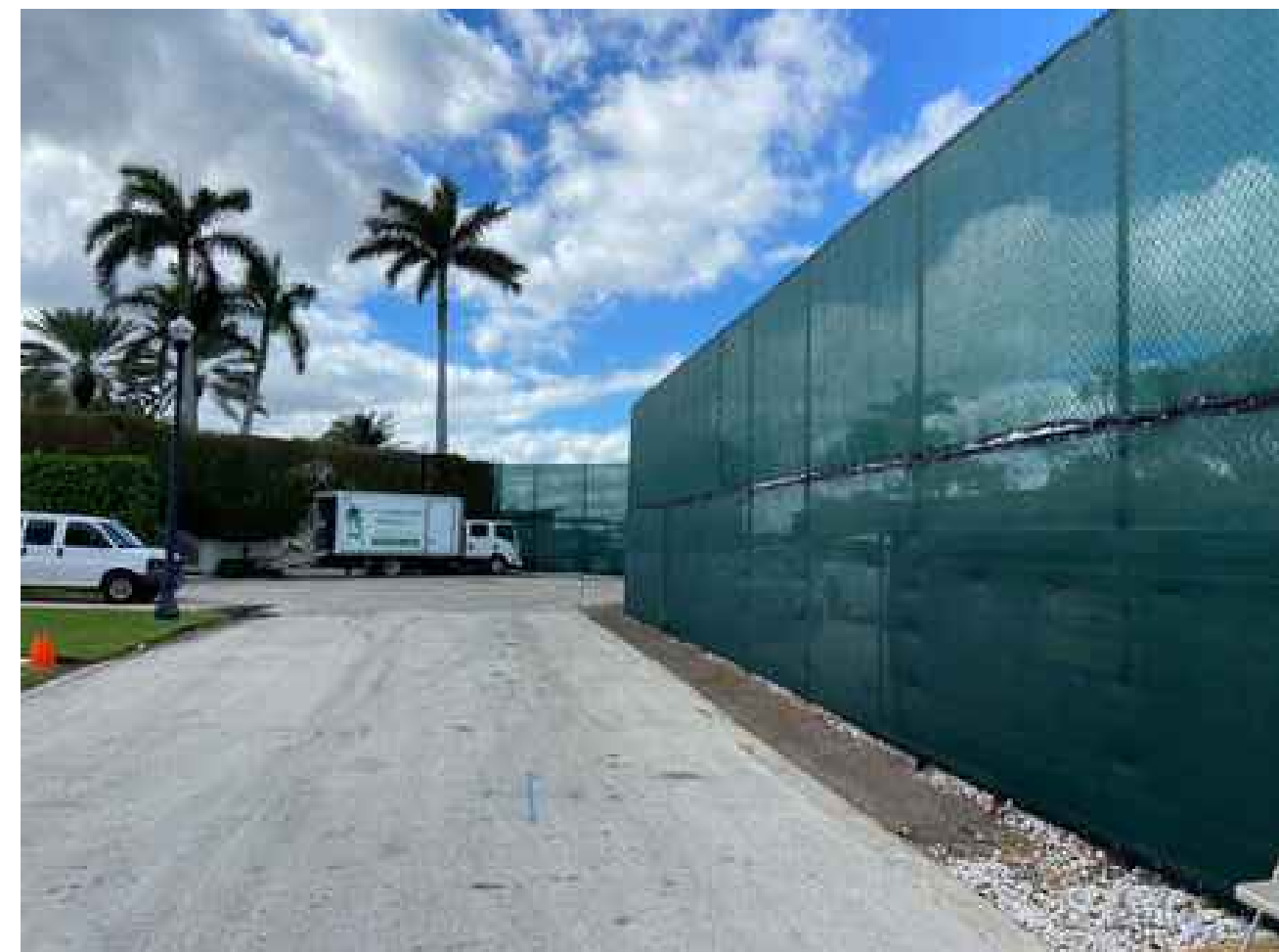
A - VIEW WEST ON VIA LINDA
