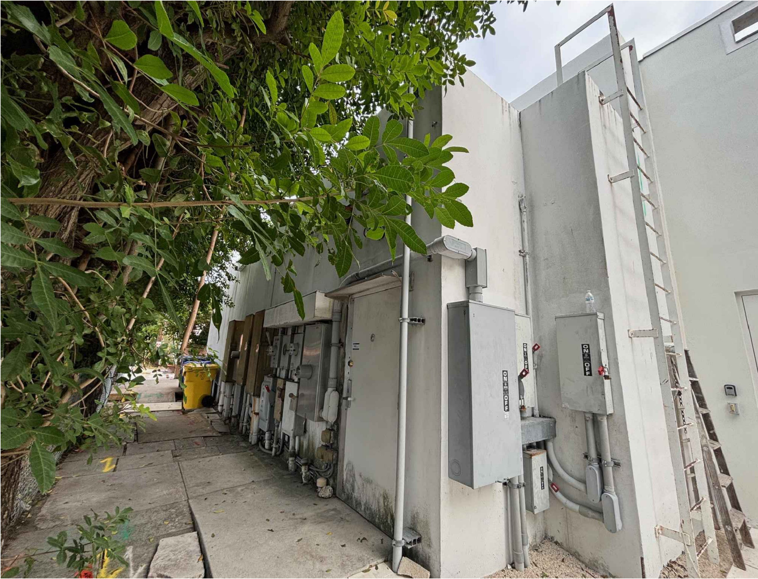
Northwest Rear Corner 221 NORTH AVE.
