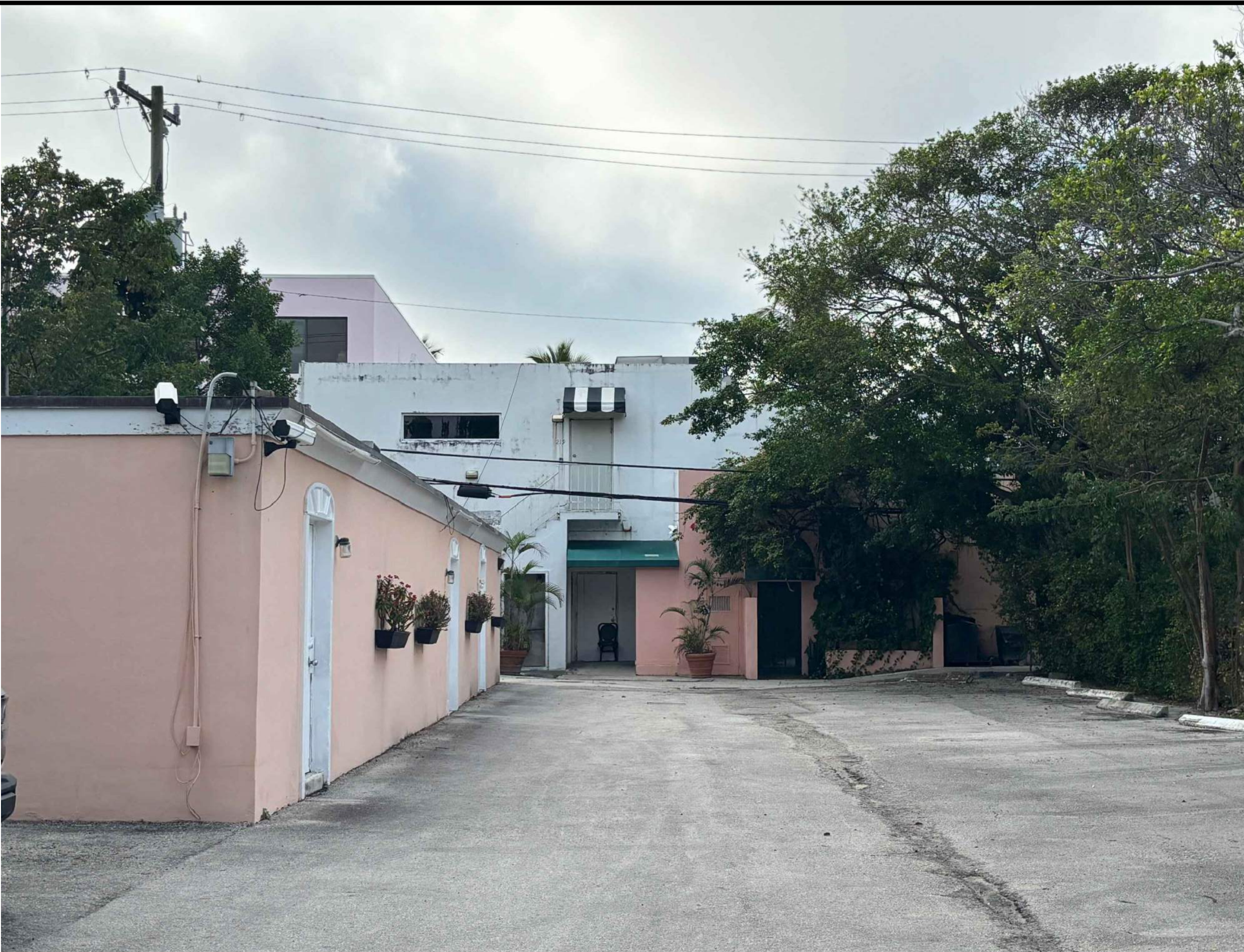
220 PERUVIAN AVE. PARKING LOT
