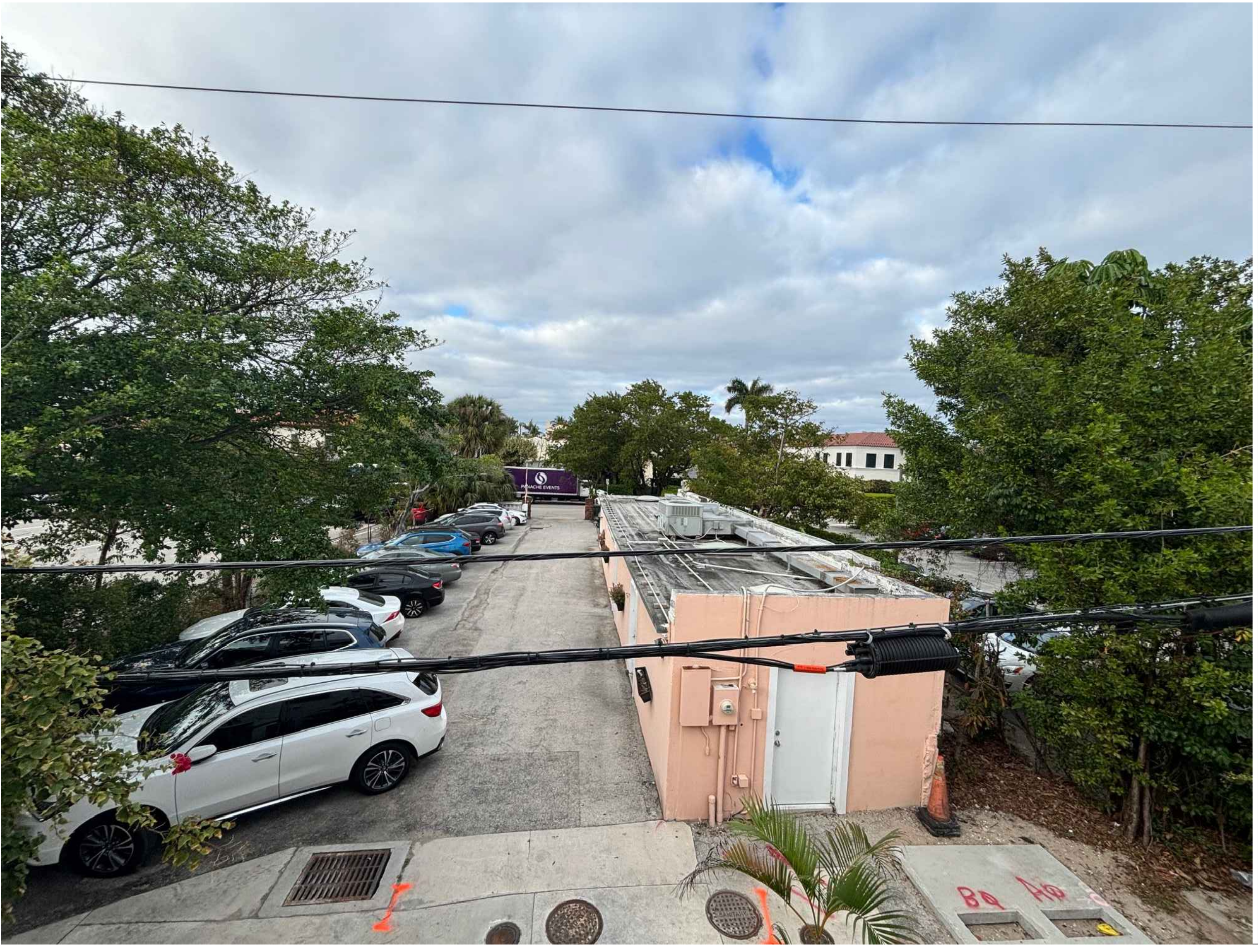
220 PERUVIAN AVE. PARKING LOT, ANNEX
