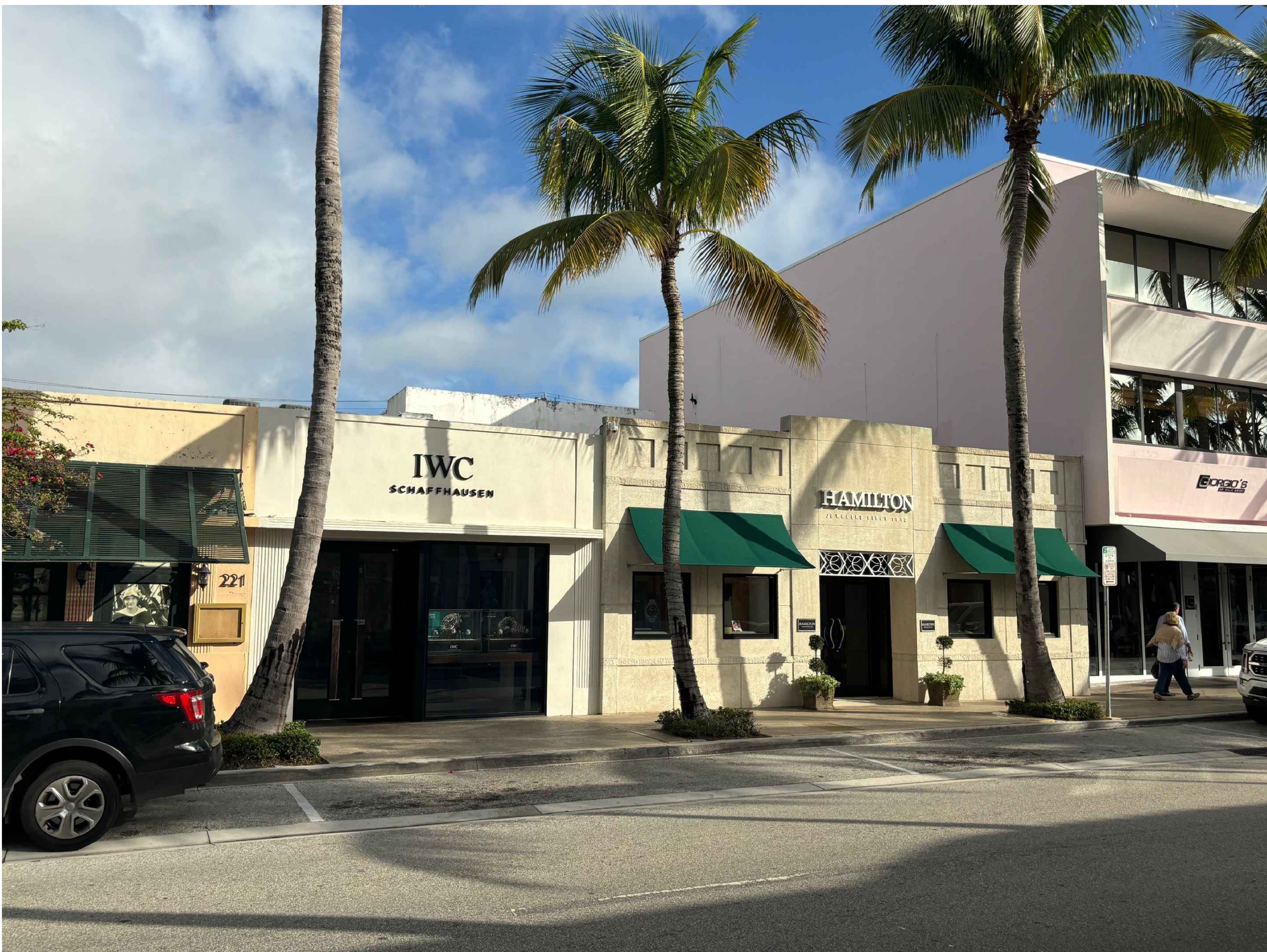
221 WORTH AVE. SUBJECT PROPERTY
