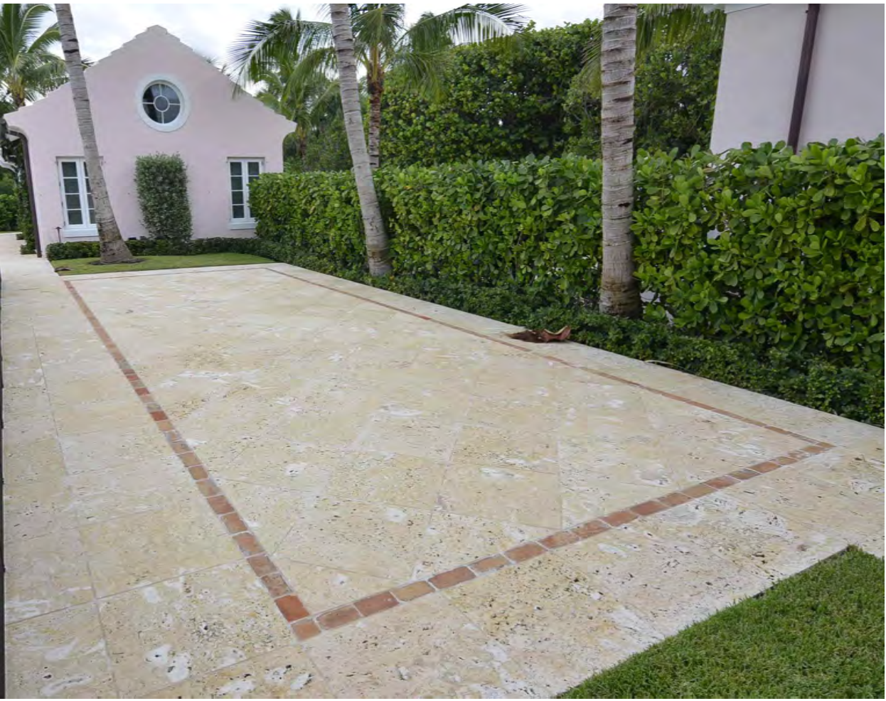
DOMINICAN SHELL STONE TERRACE WITH OLD CHICAGO BRICK INLAYS
