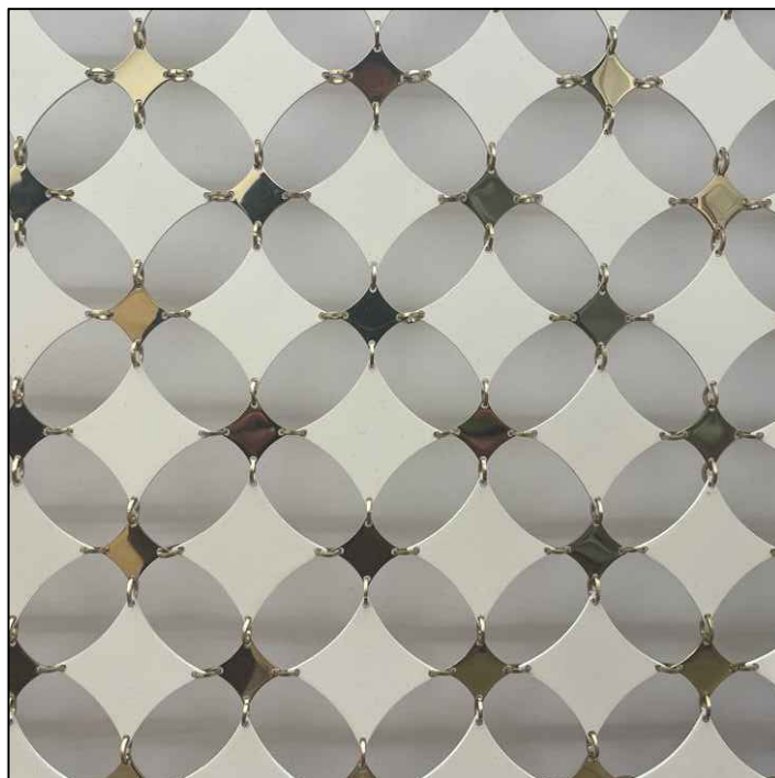
INTERIOR METAL AND LEATHER MESH, VISIBLE THROUGH GLAZING. ATTACHED TO MILLWORK BEYOND
