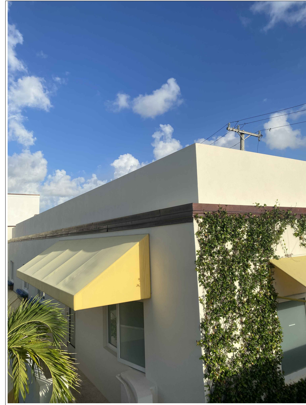
EXISTING AC SCREEN WALL @ LE BILBOQUET
