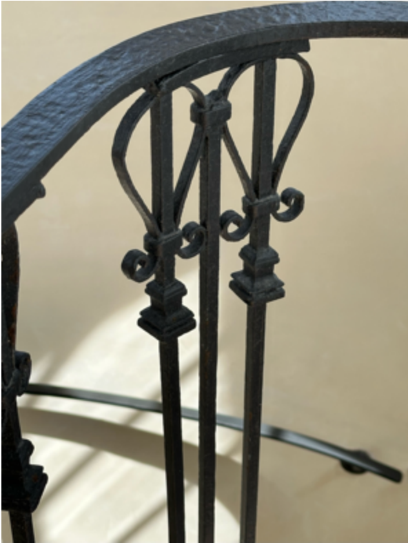
Original Wrought Iron Stair Railing Restored
