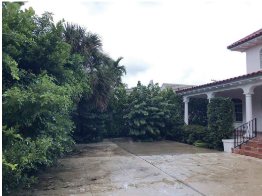
Existing Southwest Area
