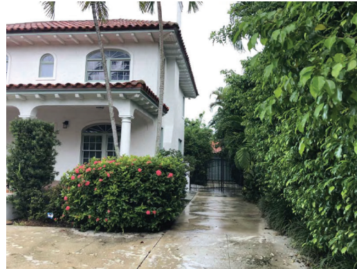
Existing North Area
