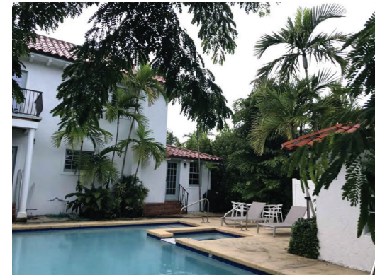
Existing Southwest Area
