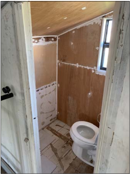
EXISTING 3RD STORY TOILET ROOM
