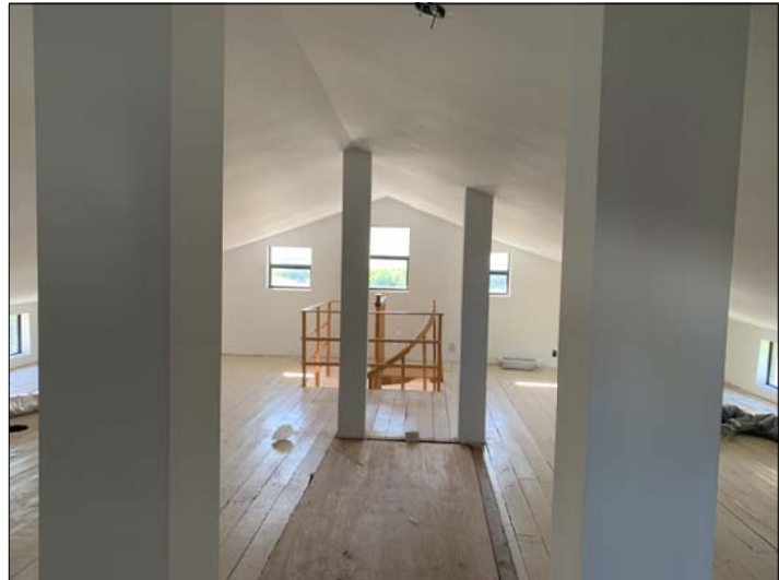
EXISTING 3RD STORY STORAGE AREA
