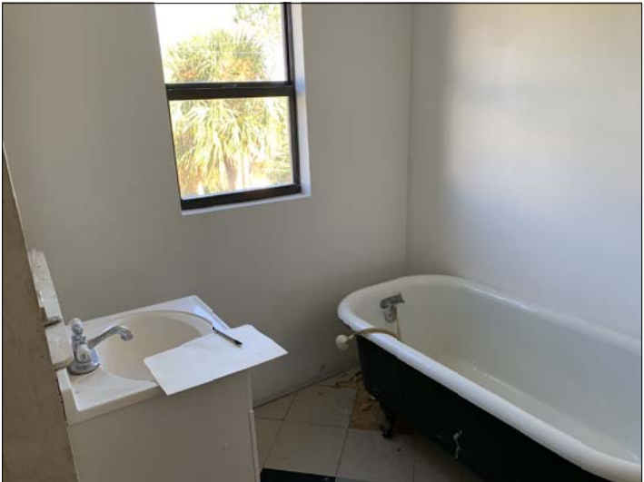
EXISTING 3RD STORY BATHROOM
