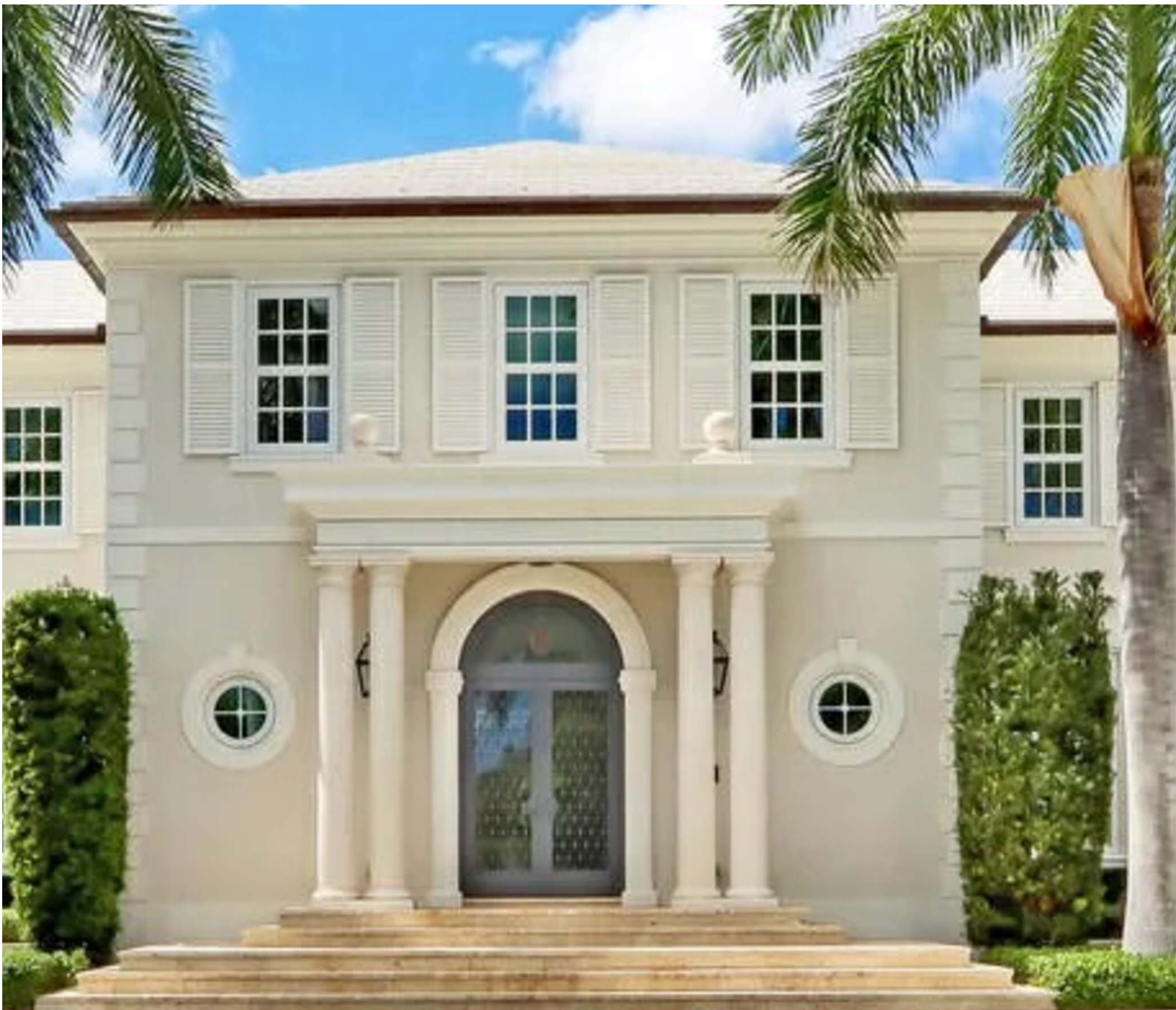
EXISTING ENTRY DOOR - EXTERIOR
