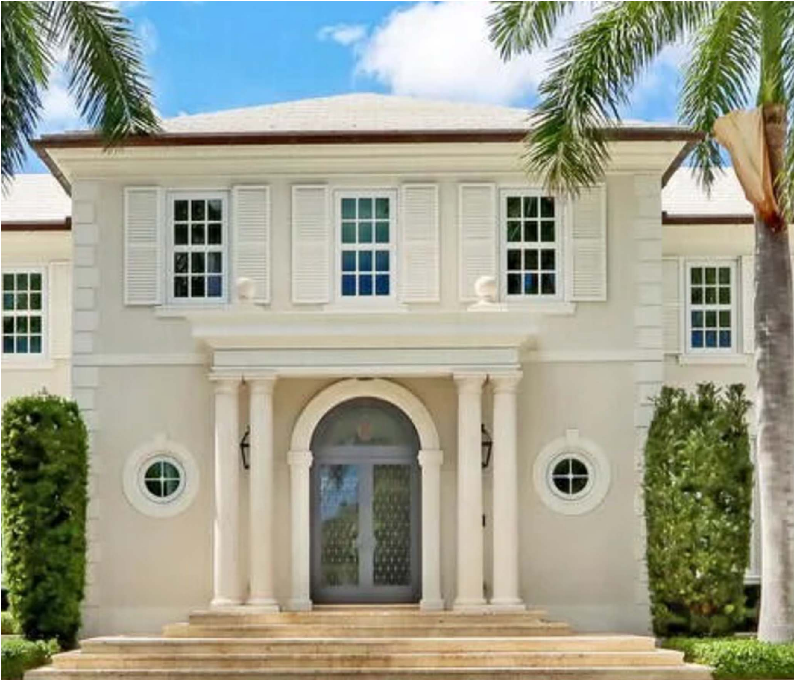
EXISTING ENTRY DOOR - EXTERIOR SCALE: 1"=1'-0"
