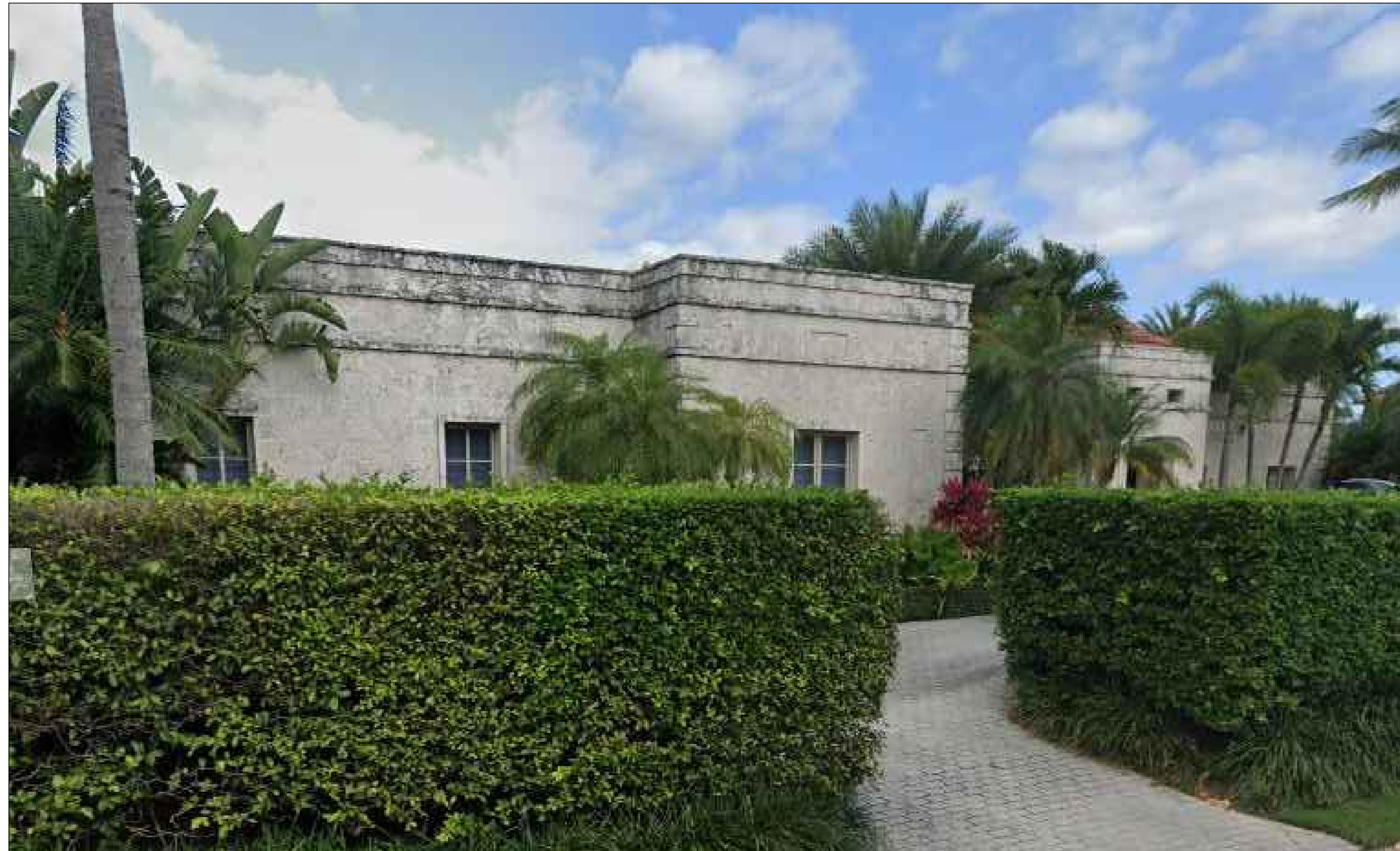
EXAMPLE OF PARAPET WITH ROOF BEHIND
