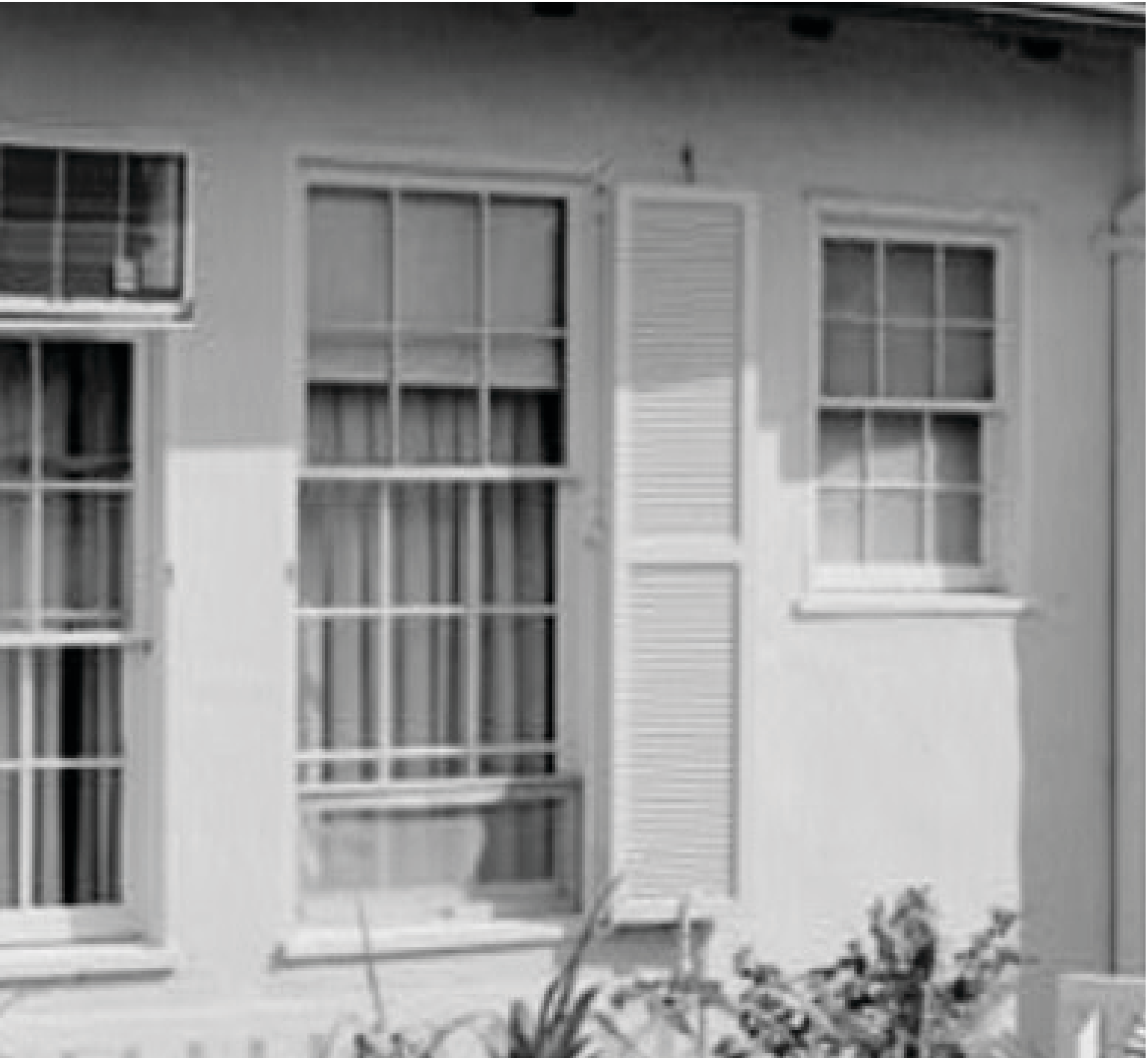
SECOND FLOOR WINDOWS (H.A.B.S. 1971)
