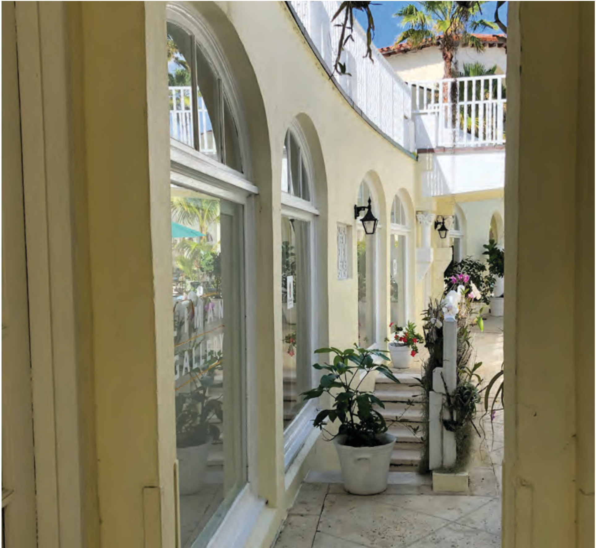
COURTYARD STOREFRONT WINDOW TODAY
