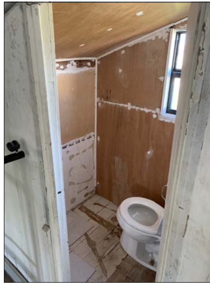
EXISTING 3RD STORY TOILET ROOM
