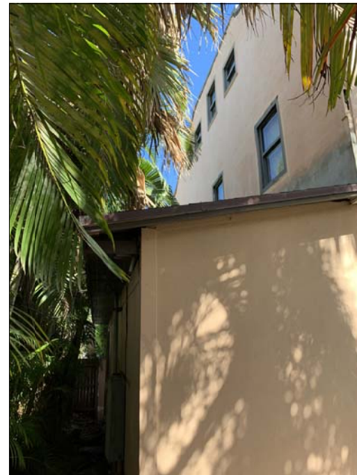
3/PH1 - WEST ELEVATION ELEVATION SUBJECT PROPERTY
