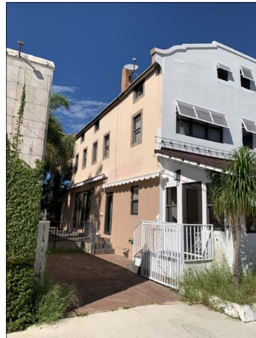
2/PH1 - WEST ELEVATION ELEVATION SUBJECT PROPERTY
