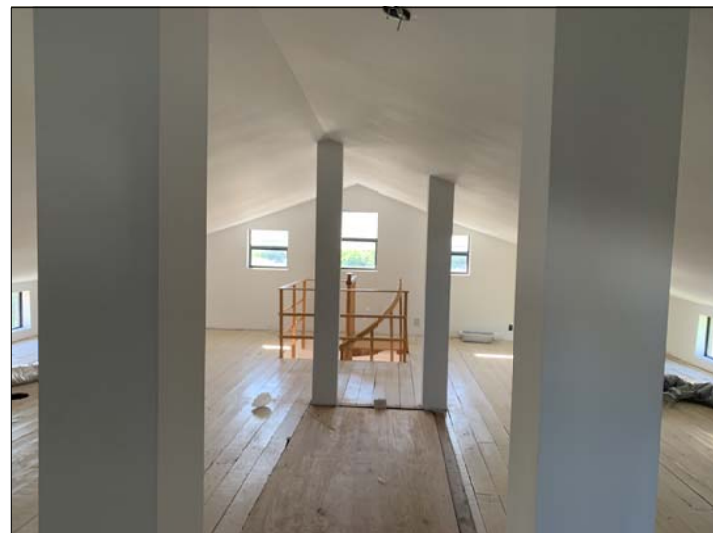
EXISTING 3RD STORY STORAGE AREA
