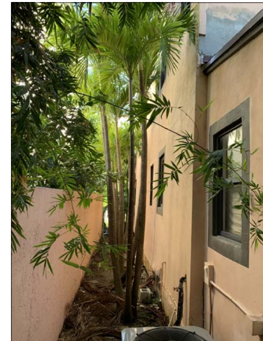
4/PH1 - WEST ELEVATION ELEVATION SUBJECT PROPERTY
