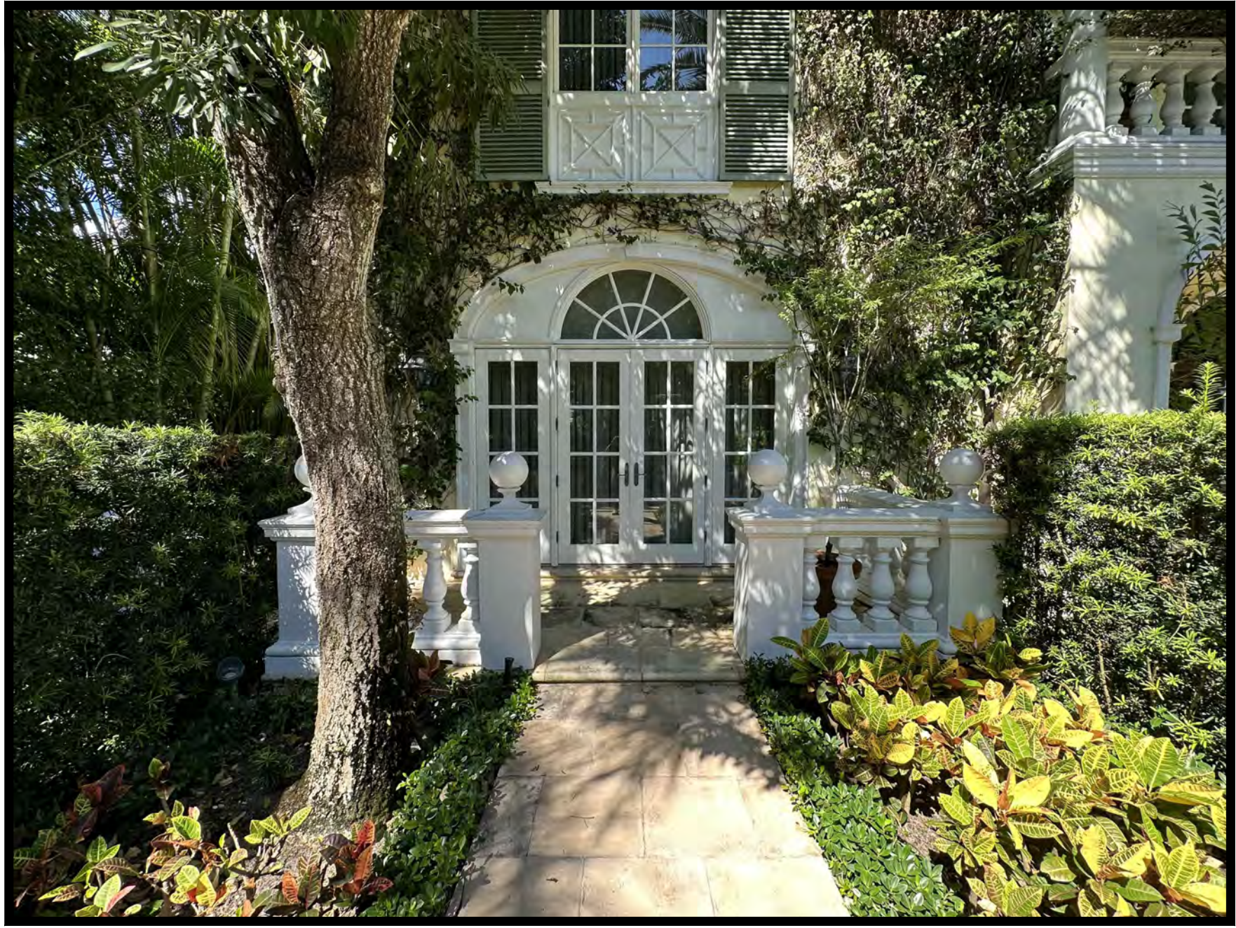
6. EXISTING EXTERIOR TERRACE
