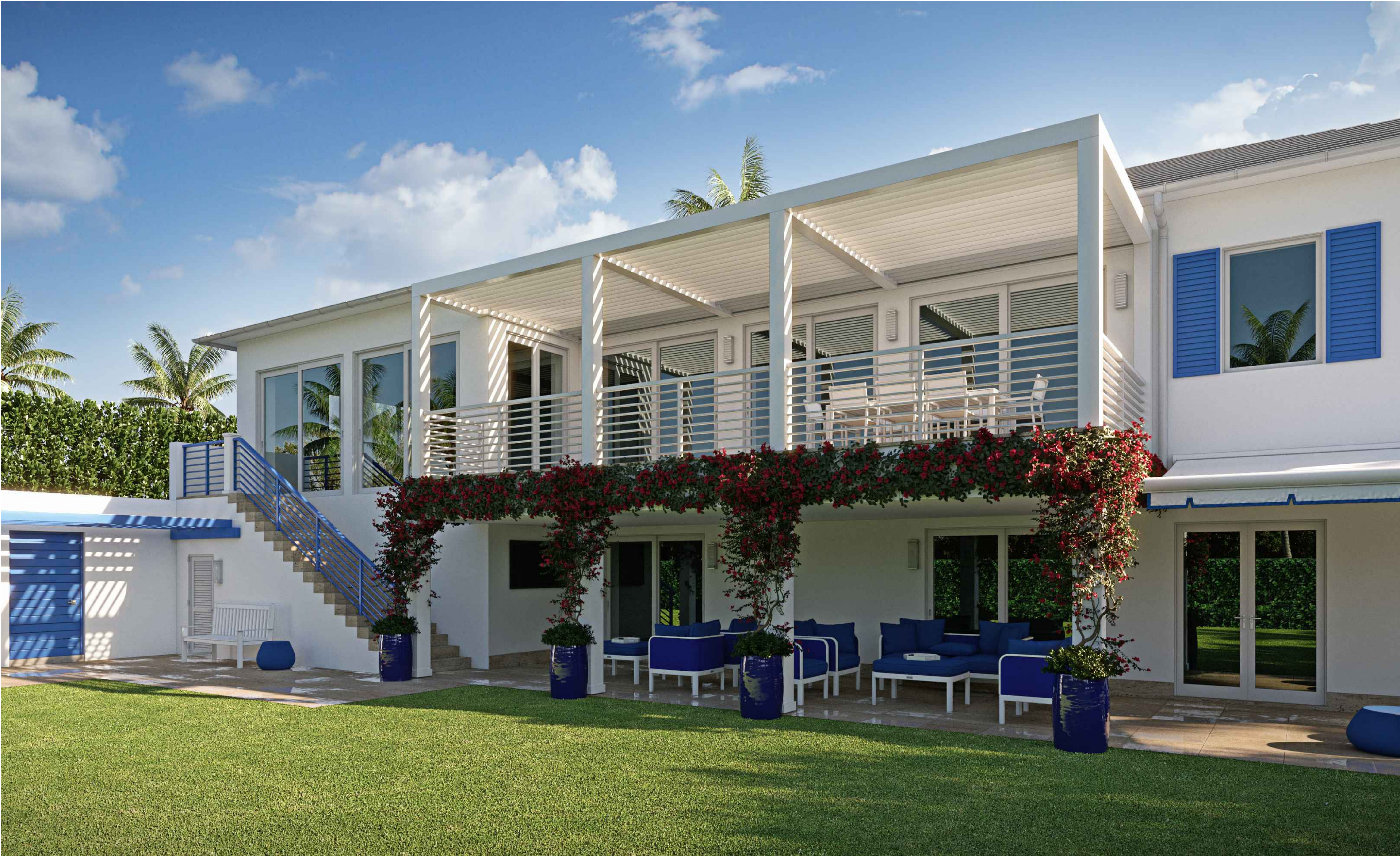
View from Back Yard
