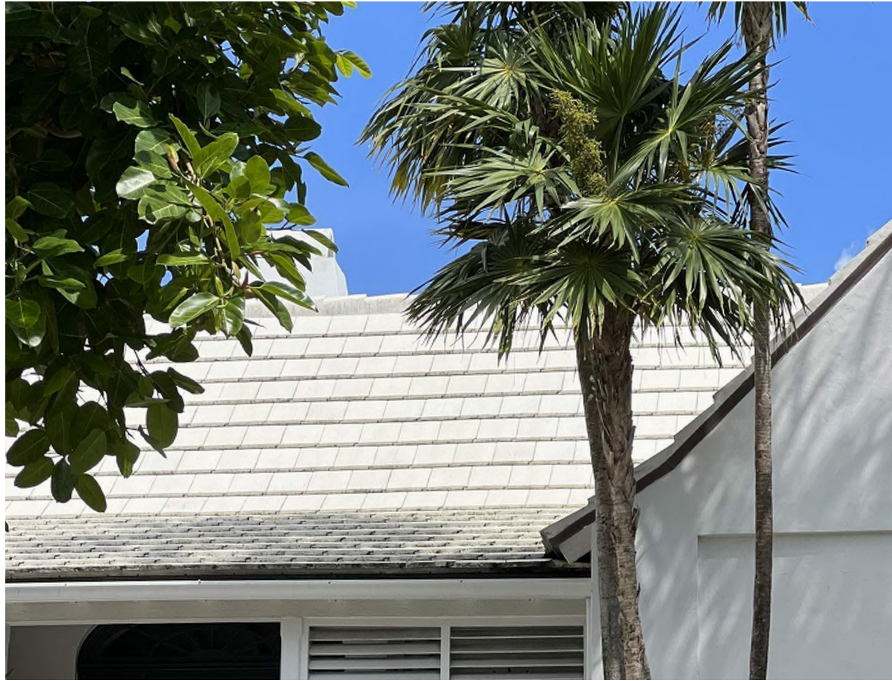
White Concrete Tile Roof, Copper Gutters
