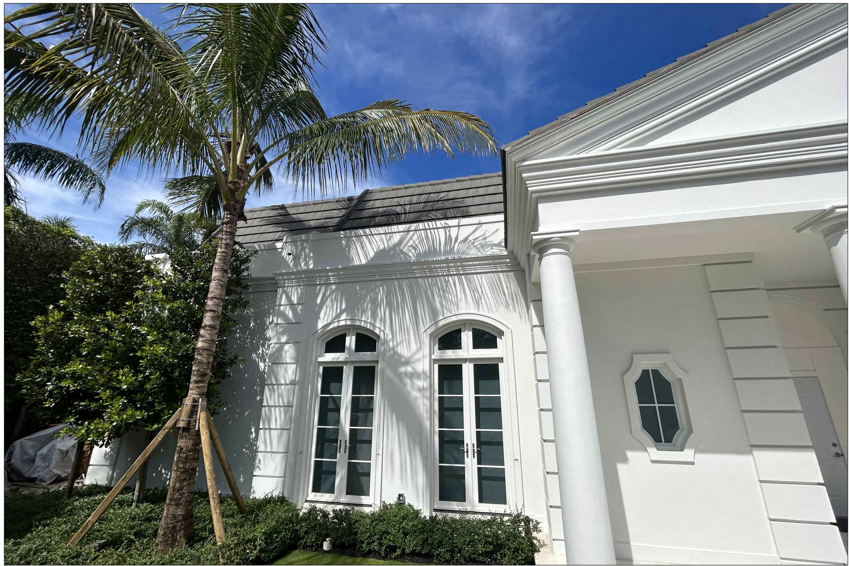
125 WELLS ROAD FRONT ENTRY- WEST
