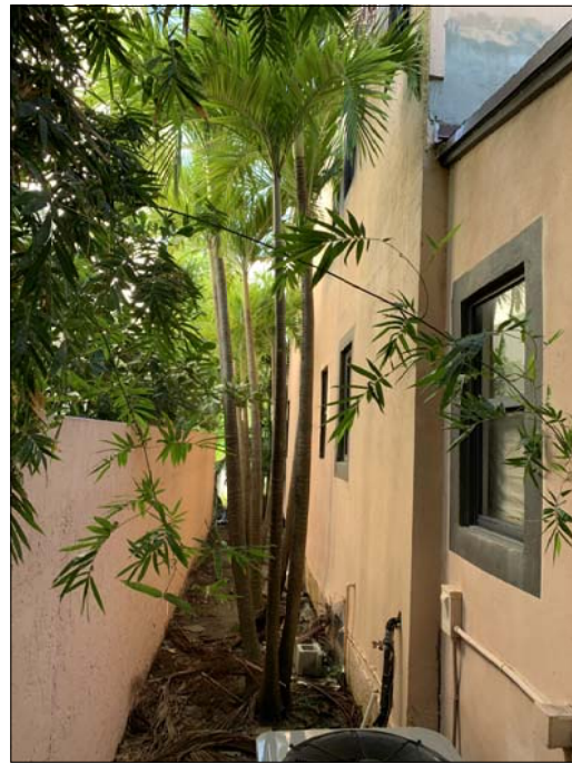
4/PH1 - WEST ELEVATION ELEVATION SUBJECT PROPERTY
