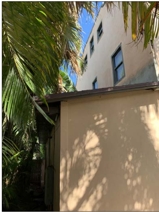
3/PH1 - WEST ELEVATION ELEVATION SUBJECT PROPERTY
