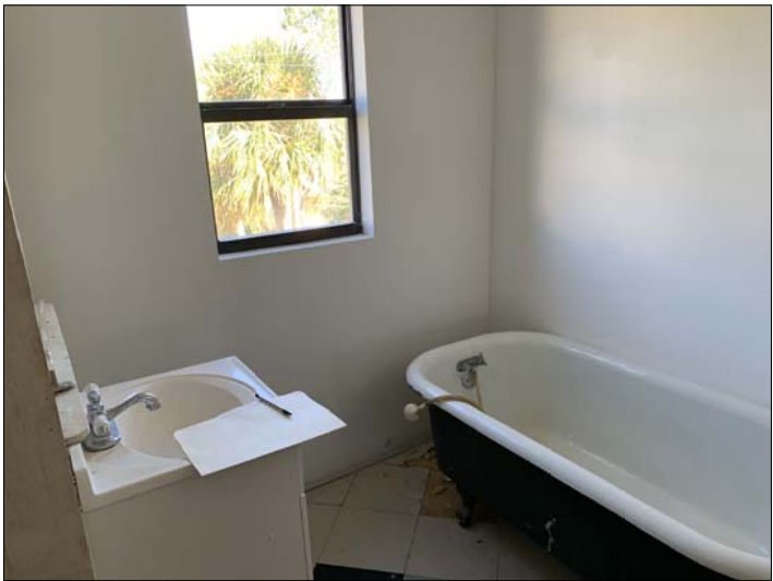
EXISTING 3RD STORY BATHROOM
