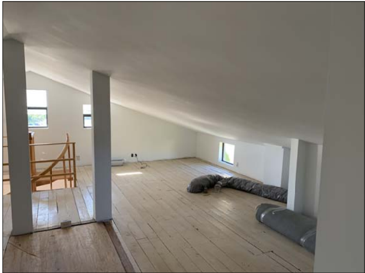
EXISTING 3RD STORY STORAGE AREA
