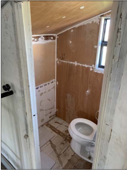
EXISTING 3RD STORY TOILET ROOM
