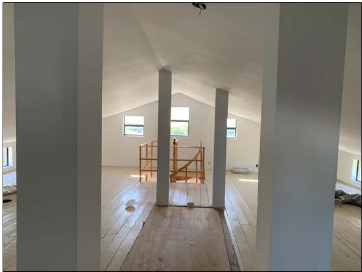
EXISTING 3RD STORY STORAGE AREA
