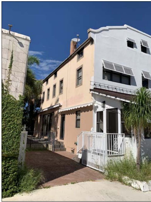
2/PH1 - WEST ELEVATION ELEVATION SUBJECT PROPERTY
