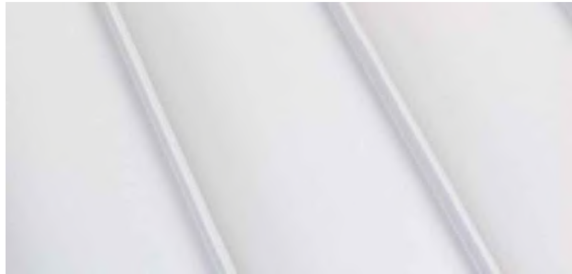
LOW SLOPE METAL ROOF
