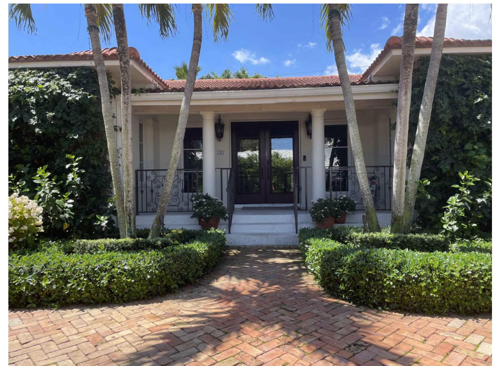
3- EXISTING COVERED ENTRY AT SOUTH ELEVATION
