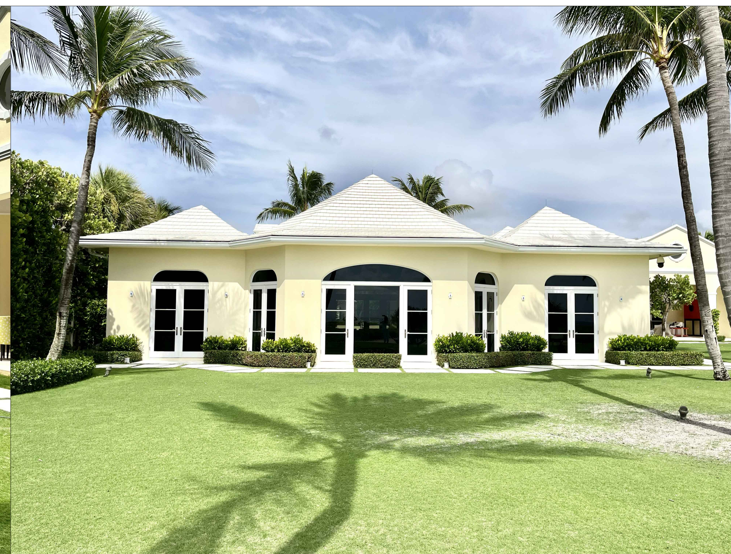
EAST SIDE EXISTING BUILDING B
