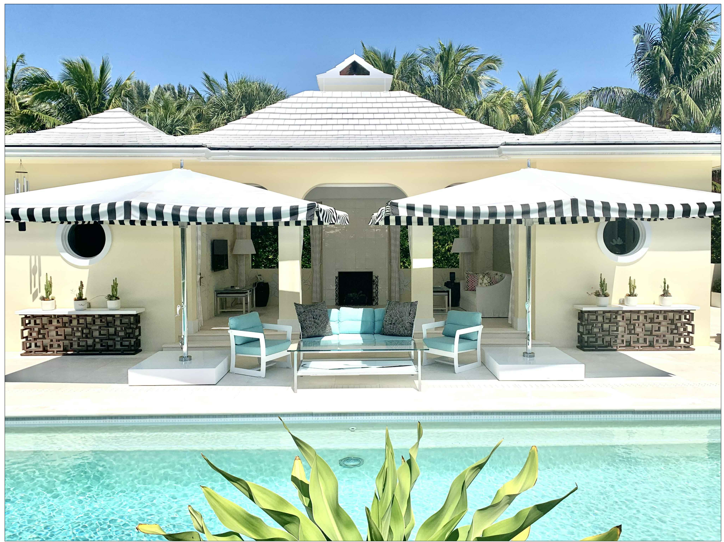
SOUTH SIDE EXISTING POOL HOUSE
