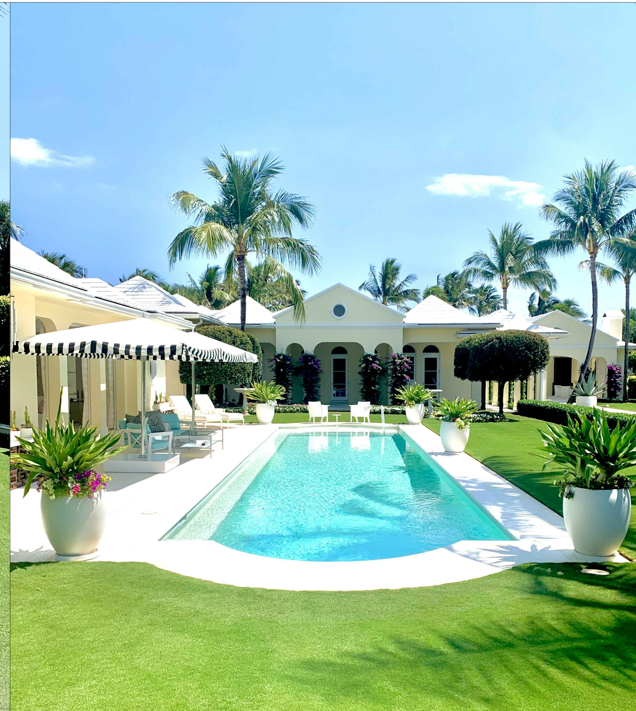
WEST SIDE EXISTING FRONT ENTRY
