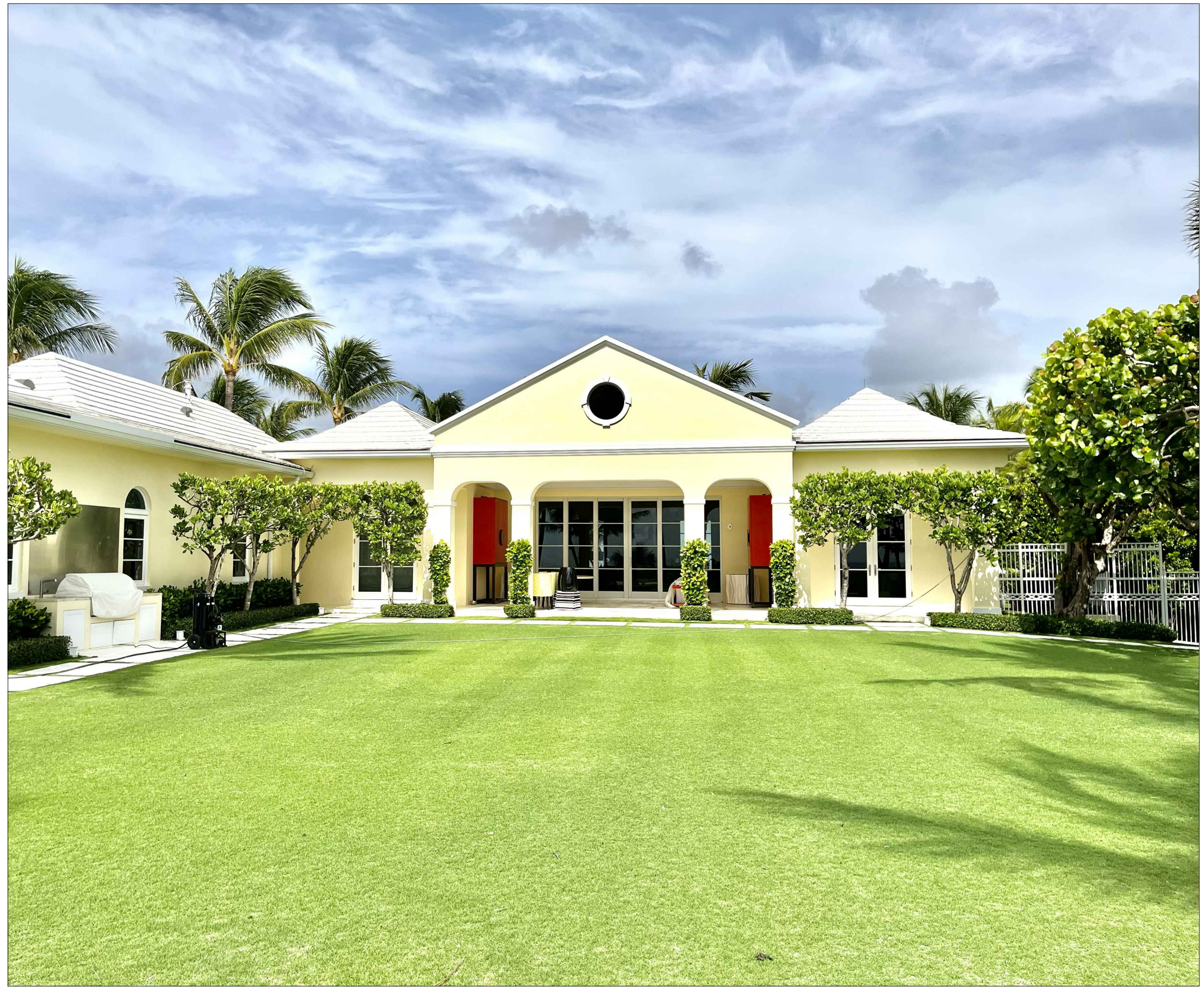
EAST SIDE EXISTING BUILDING A
