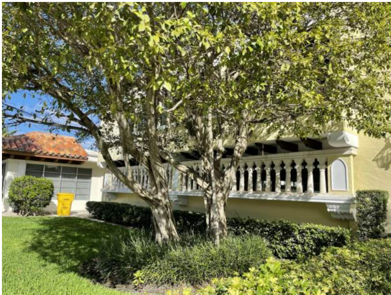
5. PARTIAL WEST FACADE
