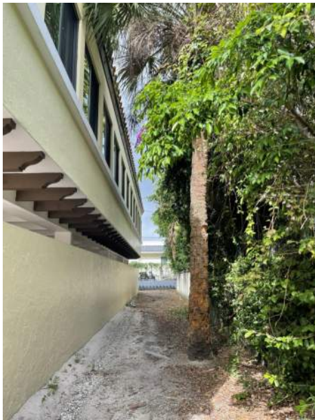
1. EAST - REAR YARD
