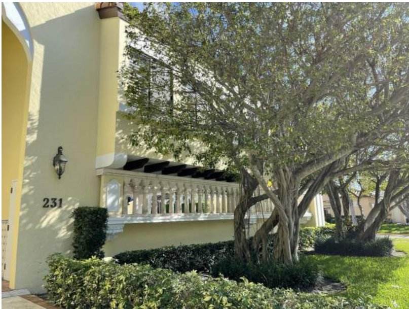
7. PARTIAL WEST FACADE
