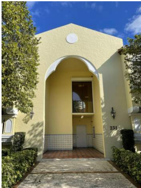
6. PARTIAL WEST FACADE
