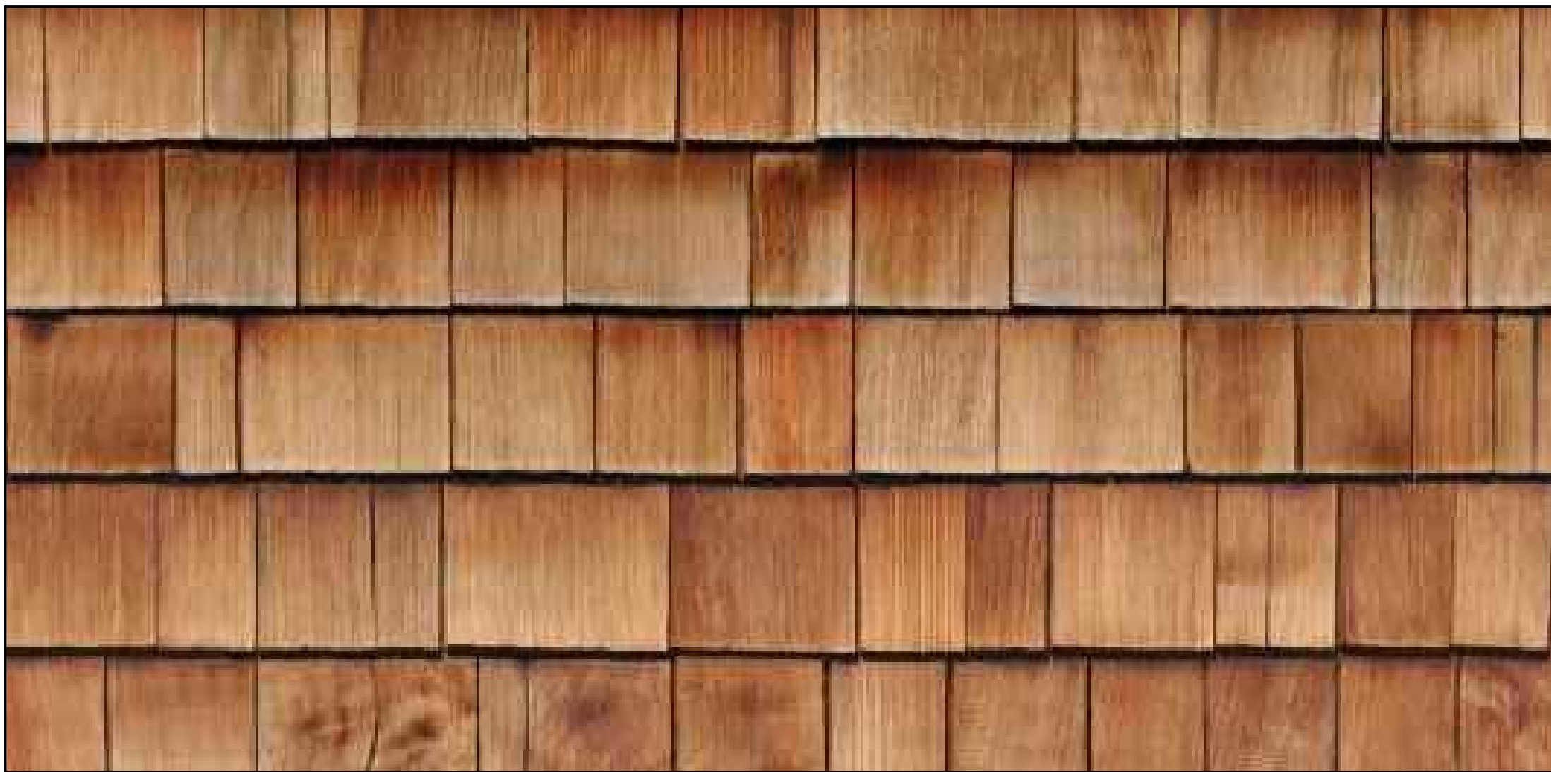
CEDAR SHAKE ROOF
