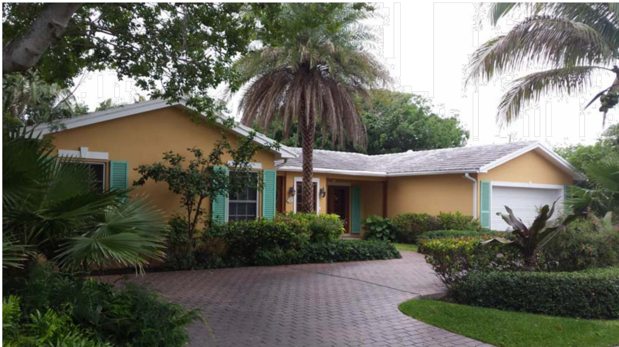
168 EAST INLET DRIVE
