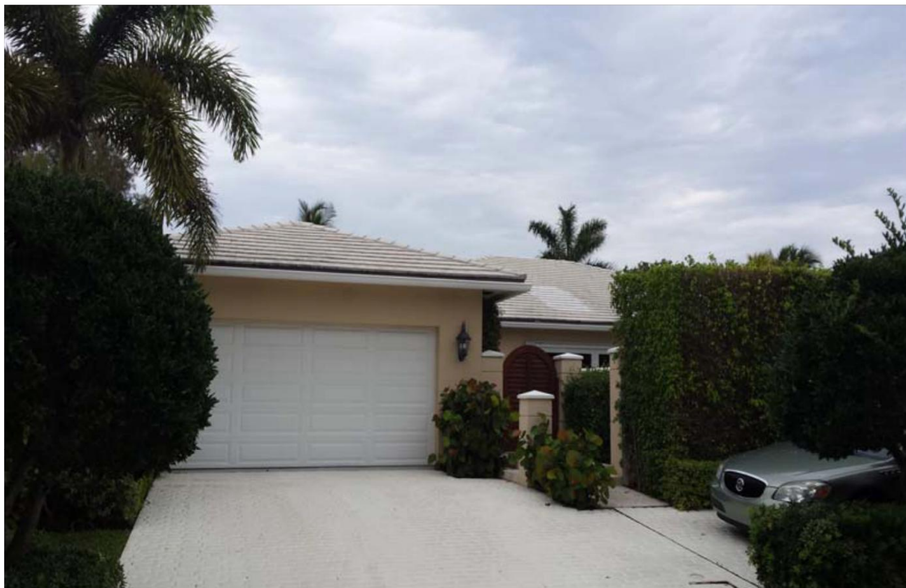
161 EAST INLET DRIVE
