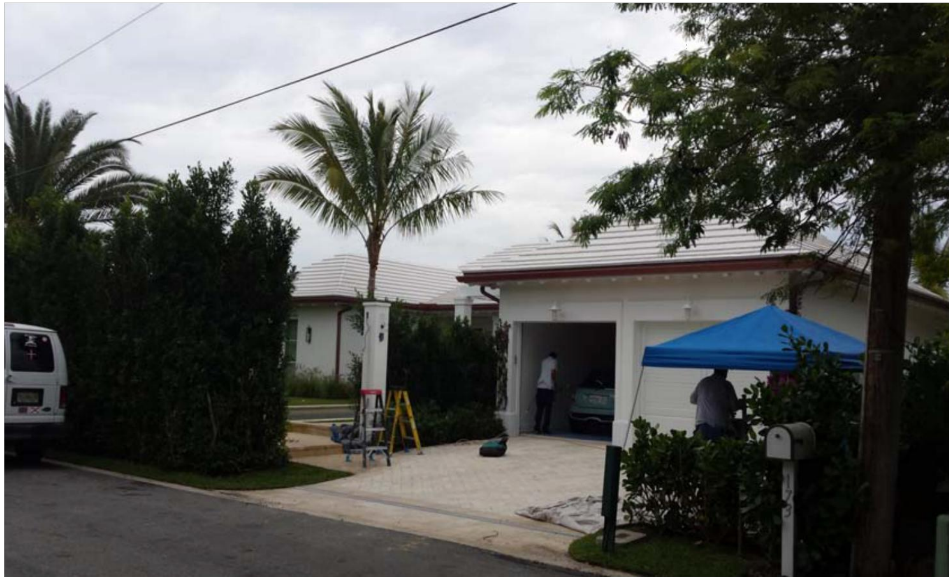
173 EAST INLET DRIVE
