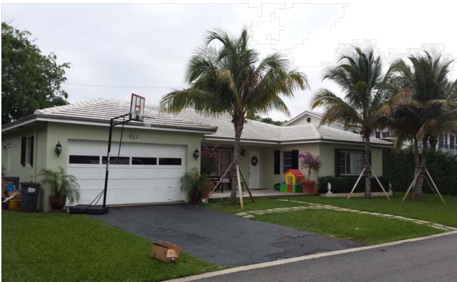
174 EAST INLET DRIVE
