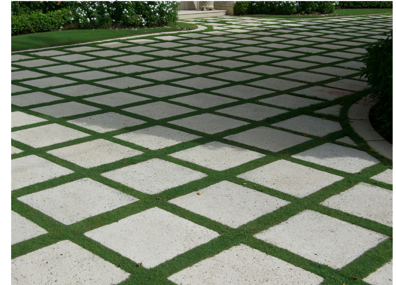
DRIVEWAY FIELD - 36" X 36" CAST STONE PAVERS W/ 6" ZOYSIA LAWN JOINTS DRIVEWAY BORDER - 12" X 24" CAST STONE PAVERS
