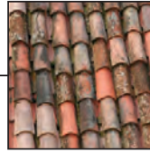
RED TILED ROOF
