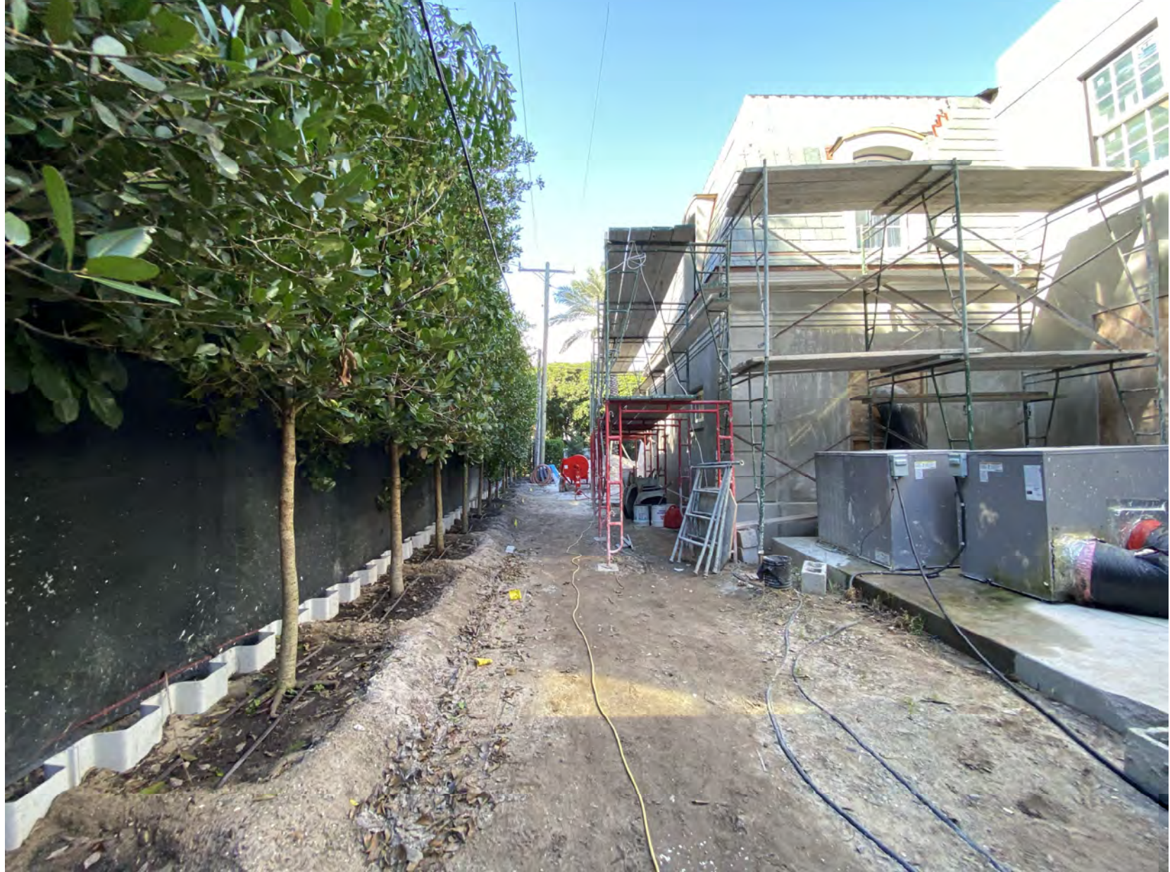
SW GATE & FENCE
