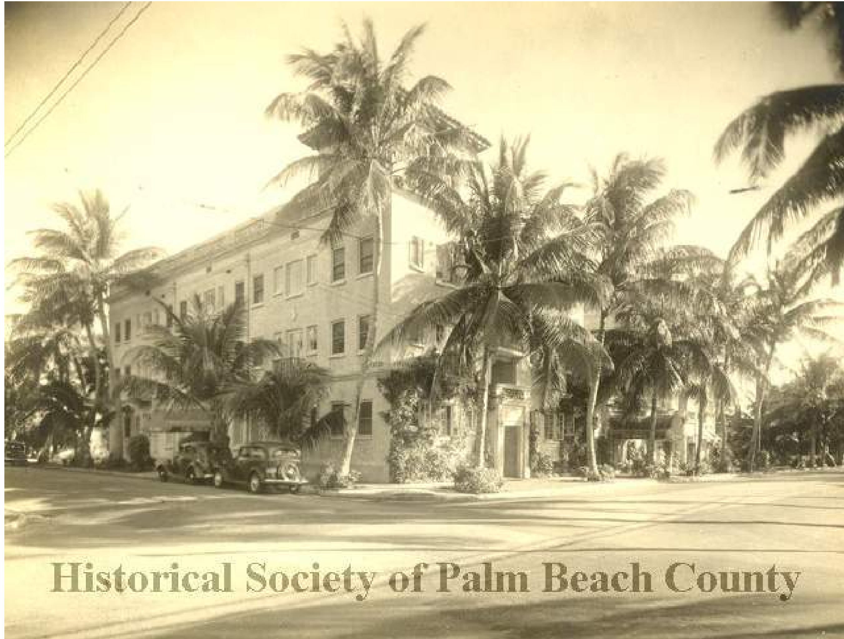
HISTORIC PHOTO (WHITE WINDOWS)
