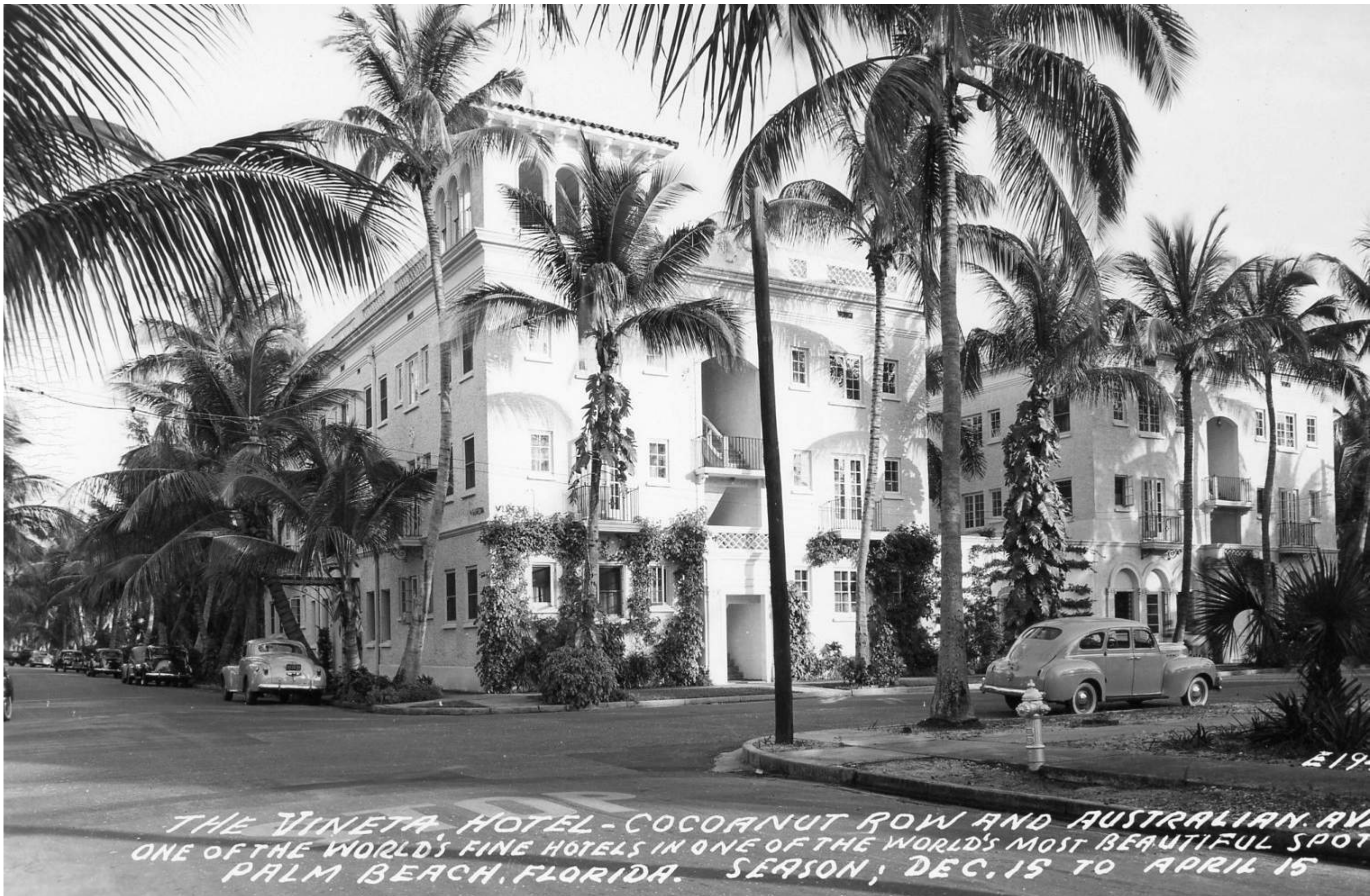
HISTORIC PHOTO (WHITE WINDOWS)
