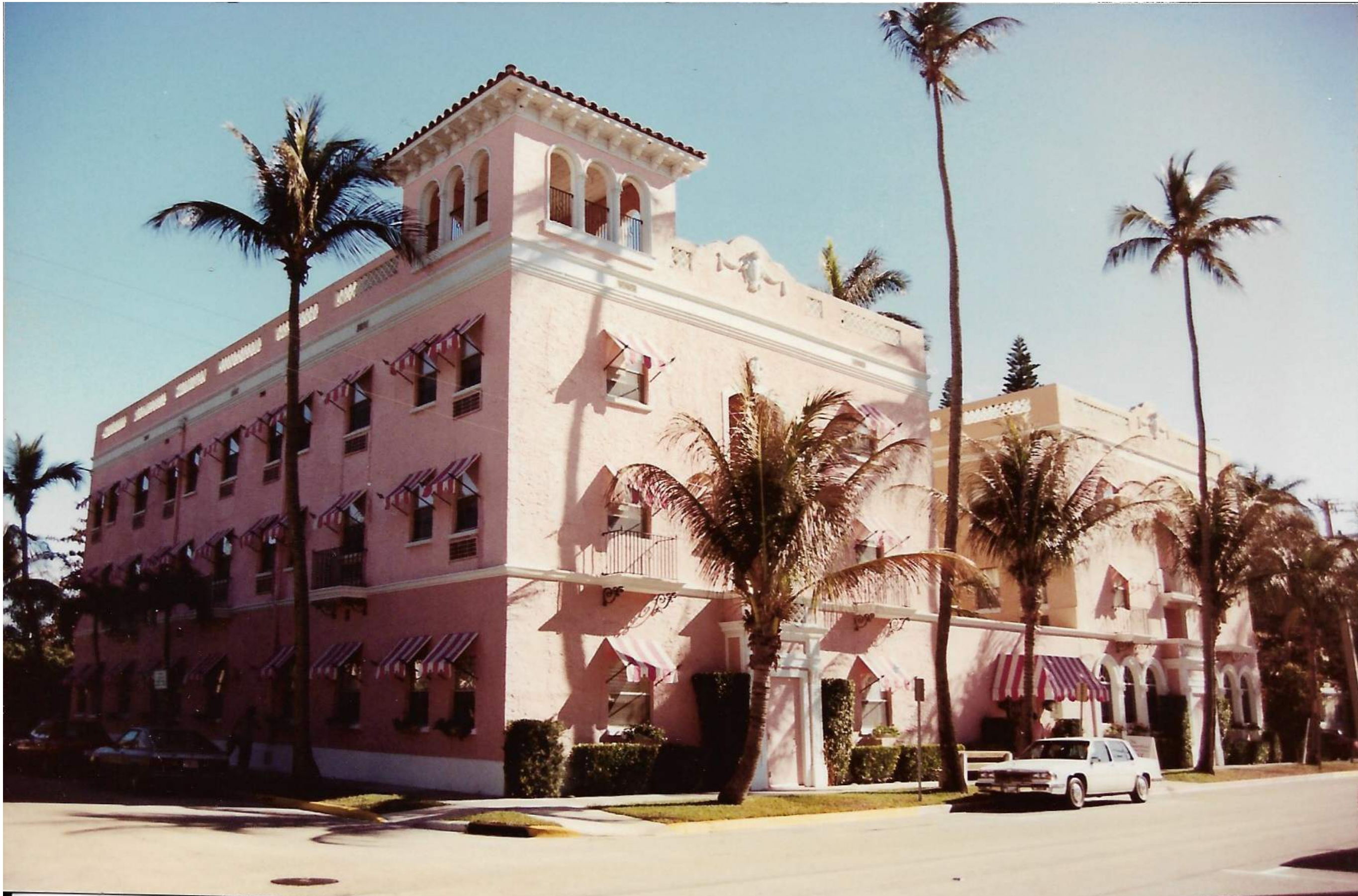
HISTORIC PHOTO (WHITE WINDOWS)
