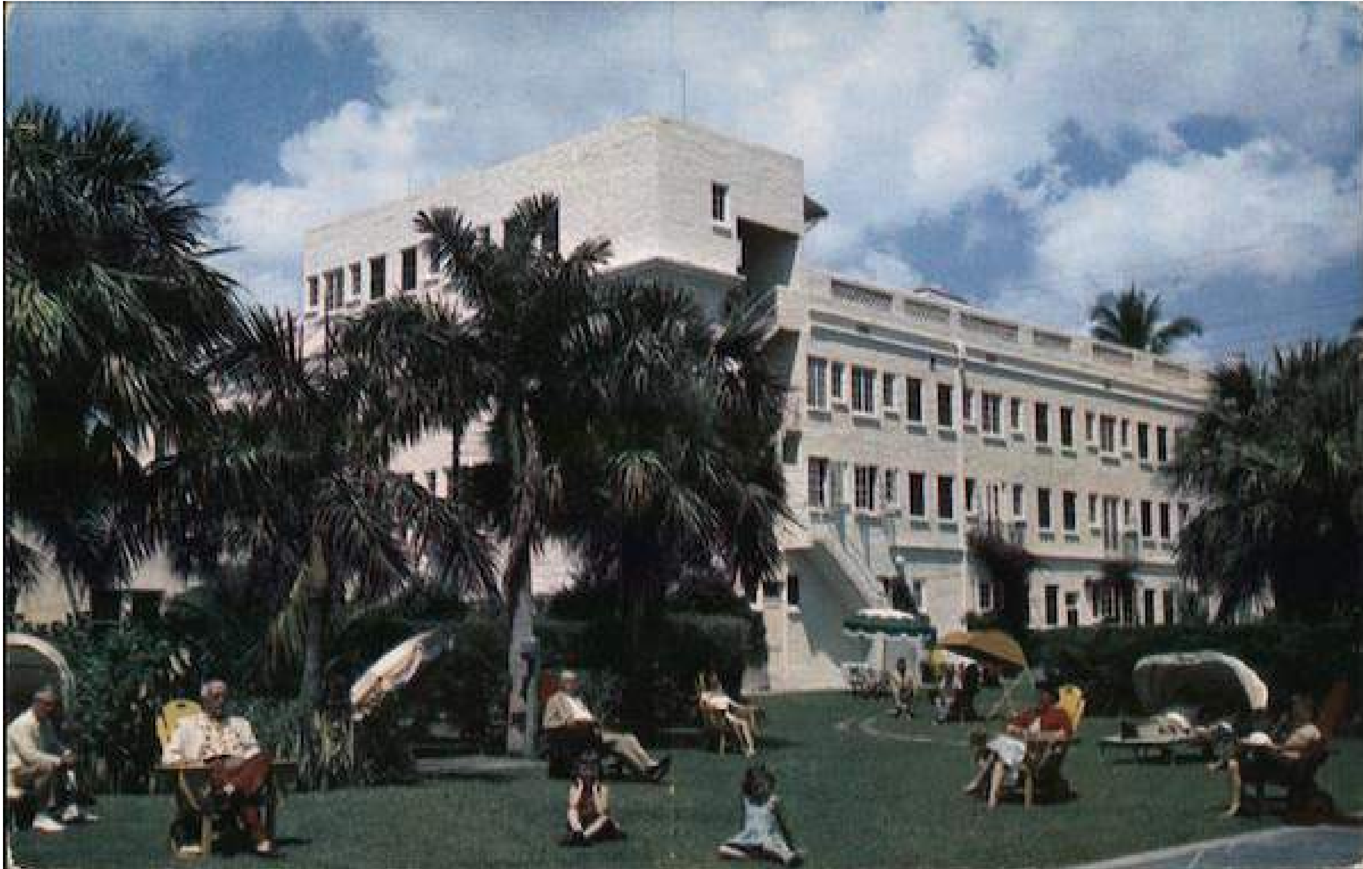
HISTORIC PHOTO (WHITE WINDOWS)
