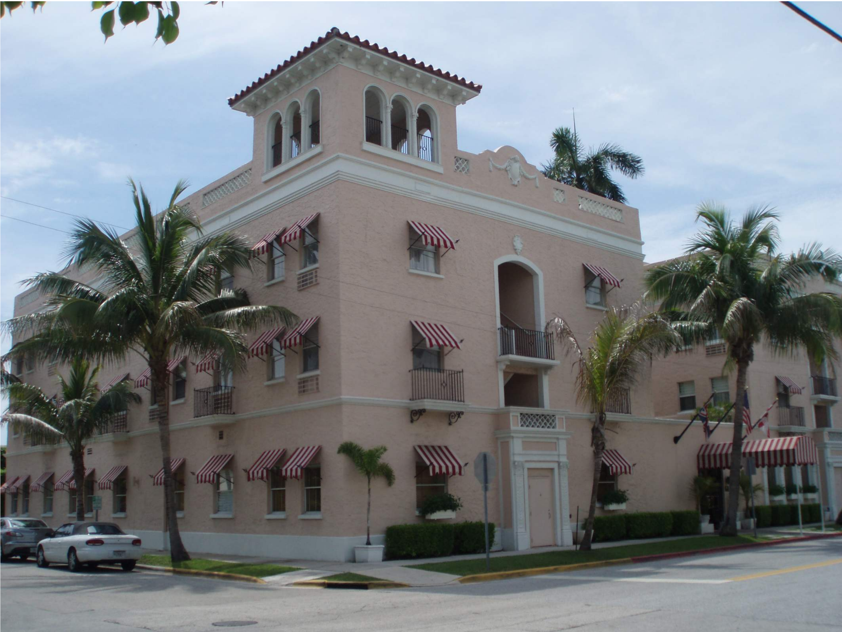
HISTORIC PHOTO (WHITE WINDOWS)
