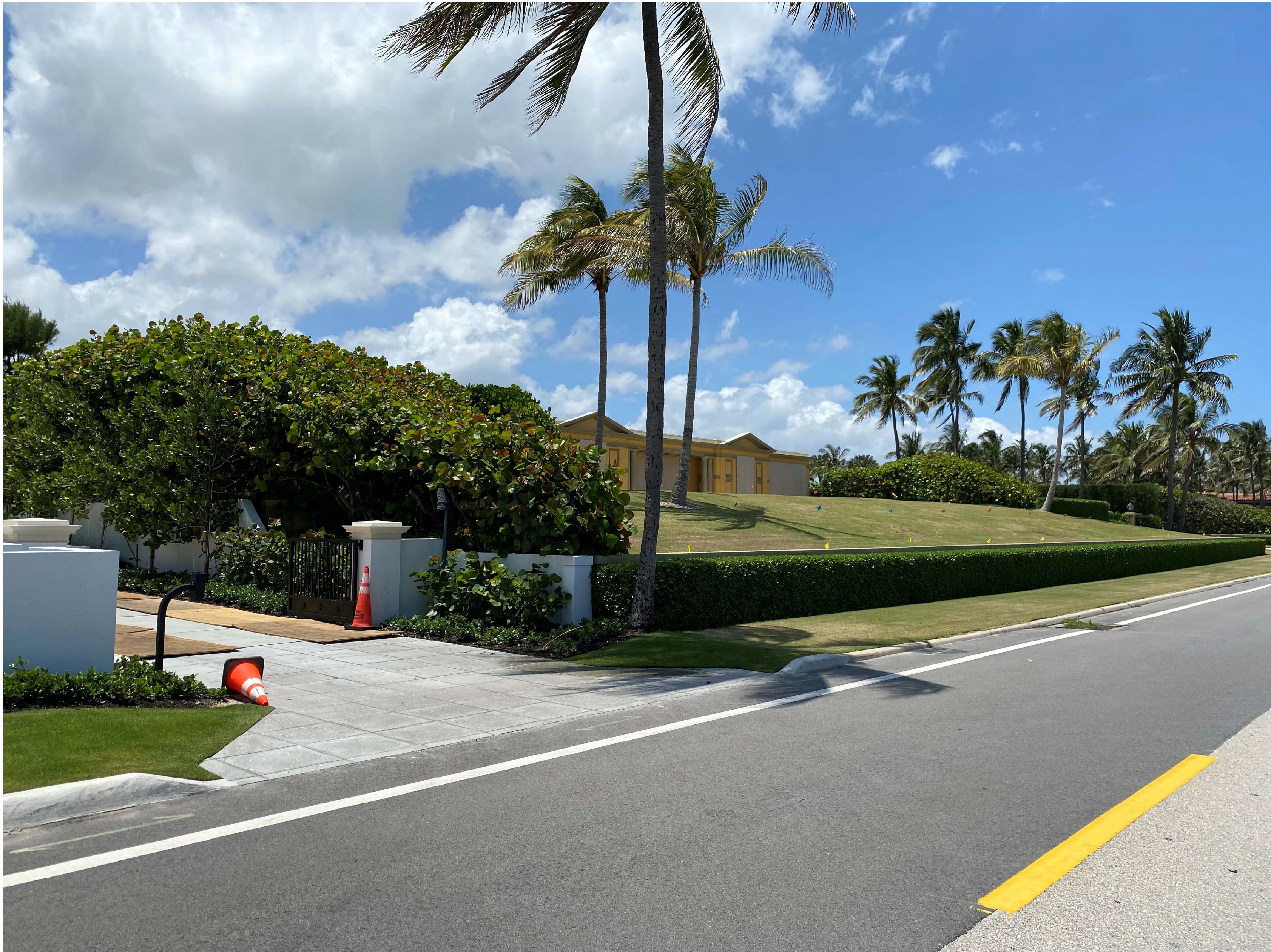
VIEW FROM SOUTH- EXISTING
