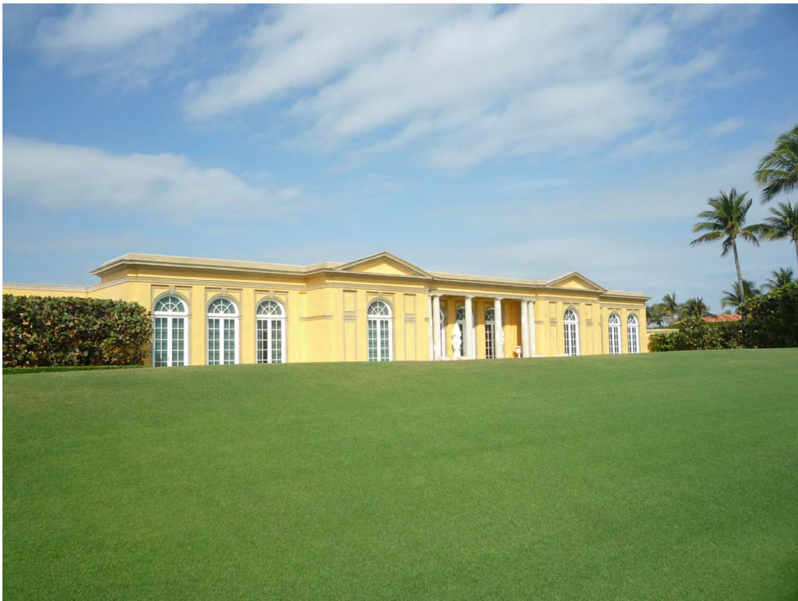
(2) EAST ELEVATION LOOKING NORTH WEST
