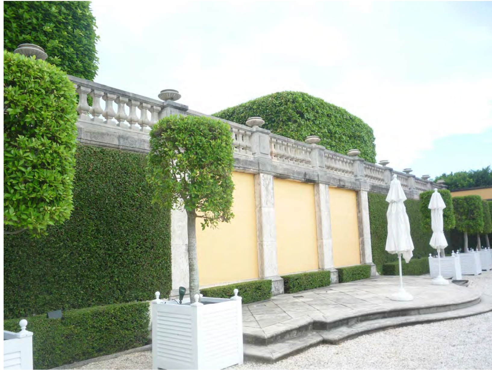
(3) WEST TERRACE ELEVATION LOOKING SOUTH
