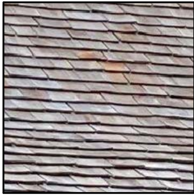
WOOD SHINGLE ROOF
